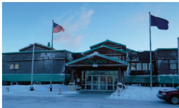
Maniiliaq Health Center, Kotzebue, Alaska
