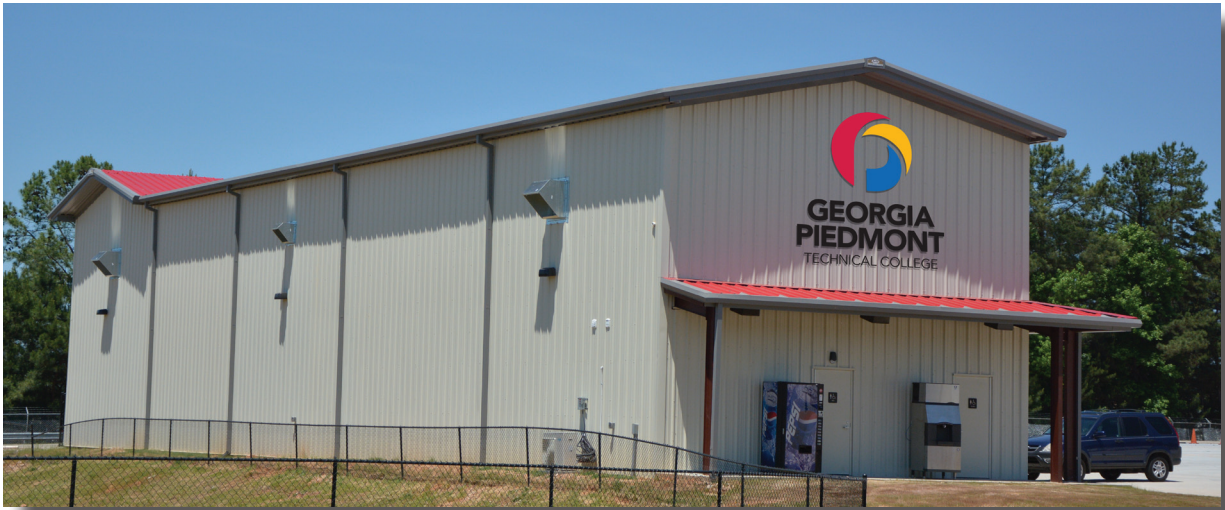
Transit Vehicle Maintenance Training Facility at GPTC's Regional Transportation Training Center in Lithonia, GA.
