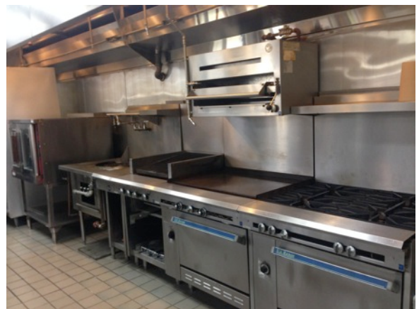
Kitchen rehab in Lauilima Building.
