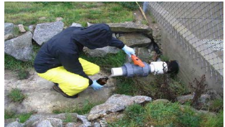
Stormwater discharges to the slot drain and is conveyed offsite through a valved pipe.
