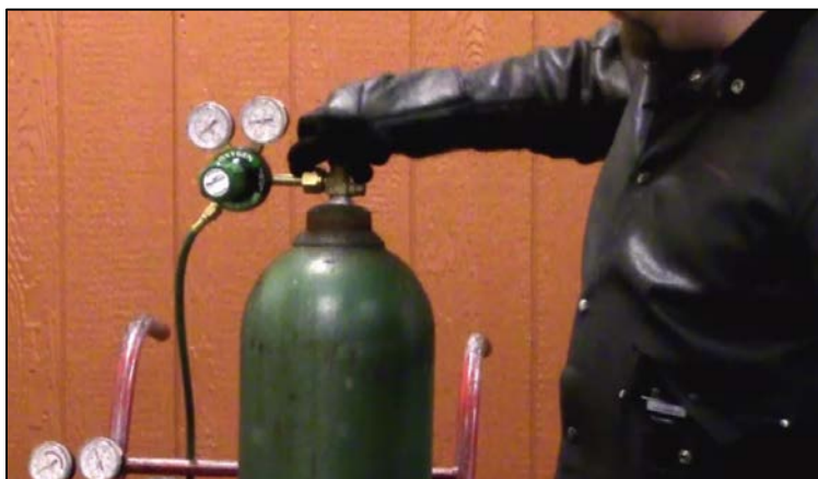
CAPTION 11. THE INSTRUCTOR TURNS THE OXYGEN VALVE OFF.
