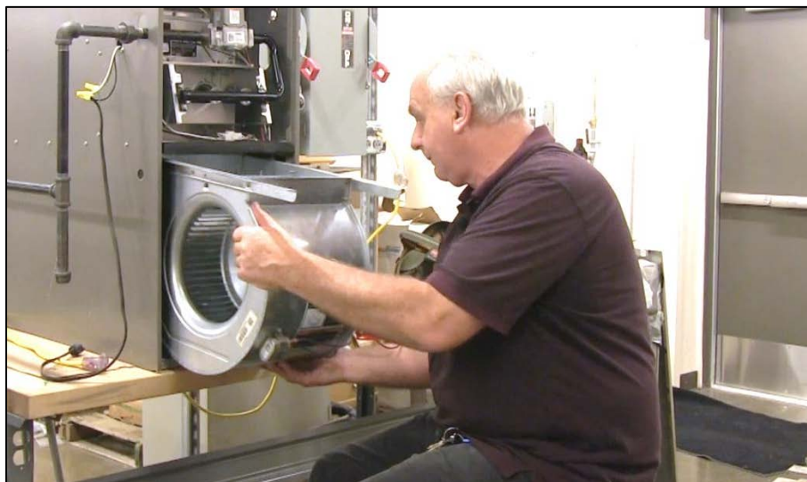
CAPTION 7. THE INSTRUCTOR RETURNS THE BLOWER MOTOR INSIDE THE FURNACE AFTER CHECKING IT.
