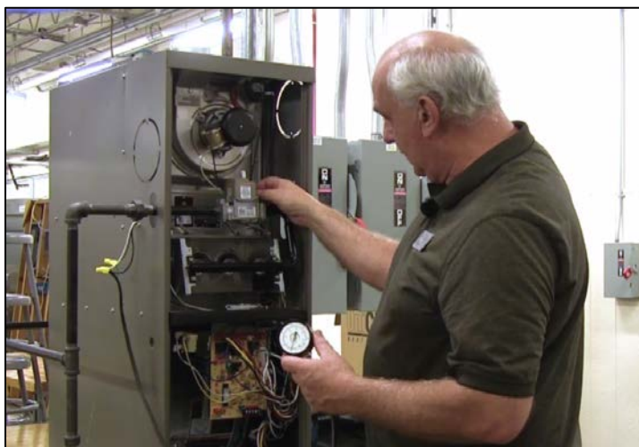
CAPTION 5. THE INSTRUCTOR TURNS OFF THE FURNACE AND IS REMOVING THE BARB FITTING FROM THE GAS VALVE.
