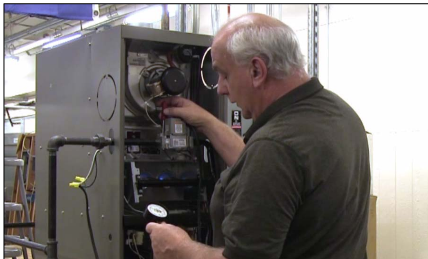
CAPTION 4. THE INSTRUCTOR TURNS THE SCREW CLOCKWISE TO INCREASE THE WATER COLUMN PRESSURE FROM 3 INCHES TO 3 ½ INCHES.
