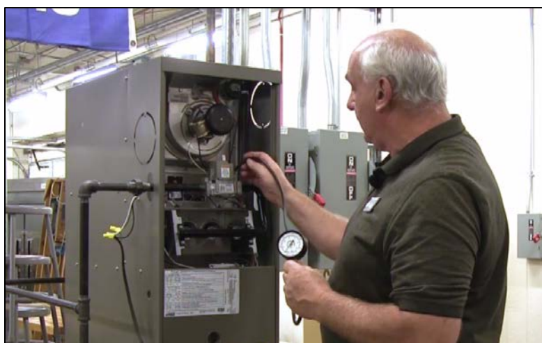
CAPTION 2. THE RUBBER HOSE OF THE WATER COLUMN GAUGE IS FITTED TO THE BARB FITTING PLACED ON THE GAS VALVE.
