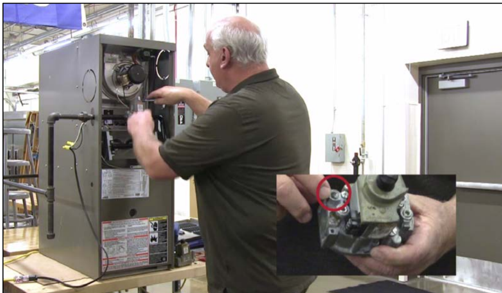
CAPTION 1. THE INSTRUCTOR IS REMOVING THE PLUG ON THE GAS VALVE.
