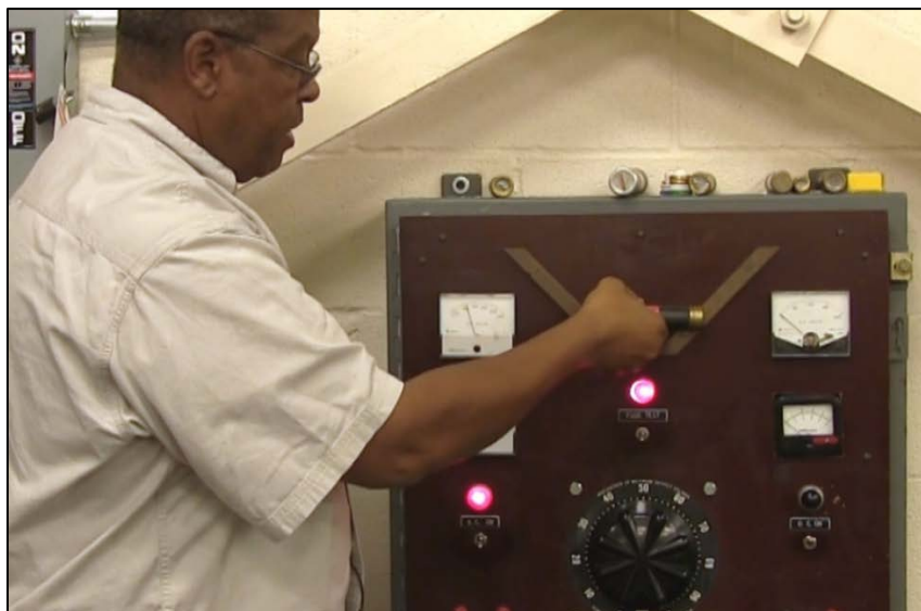
CAPTION 7. THE INSTRUCTOR TESTS A FERRULE CARTRIDGE TYPE FUSE. THE LIGHT IS ON, SIGNALLING THAT THE FUSE IS IN GOOD CONDITION AND IS WORKING PROPERLY.
