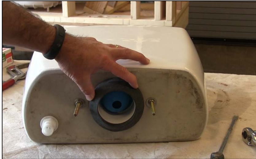
CAPTION 12. BOTTOM VIEW OF THE TOILET TANK WITH ITS INSTALLED PARTS.
