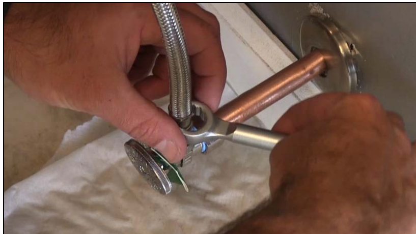
CAPTION 23. THE TOILET SUPPLY LINE IS BEING INSTALLED.
