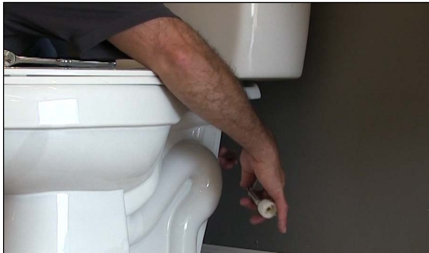
CAPTION 29. THE TOILET SUPPLY IS BEING CONNECTED TO THE FILL VALVE
