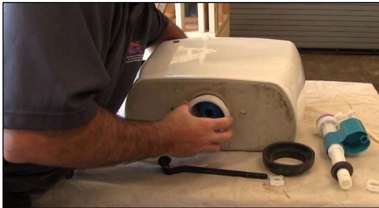
CAPTION 4. THE INSTRUCTOR INSTALLING THE FLUSH VALVE.
