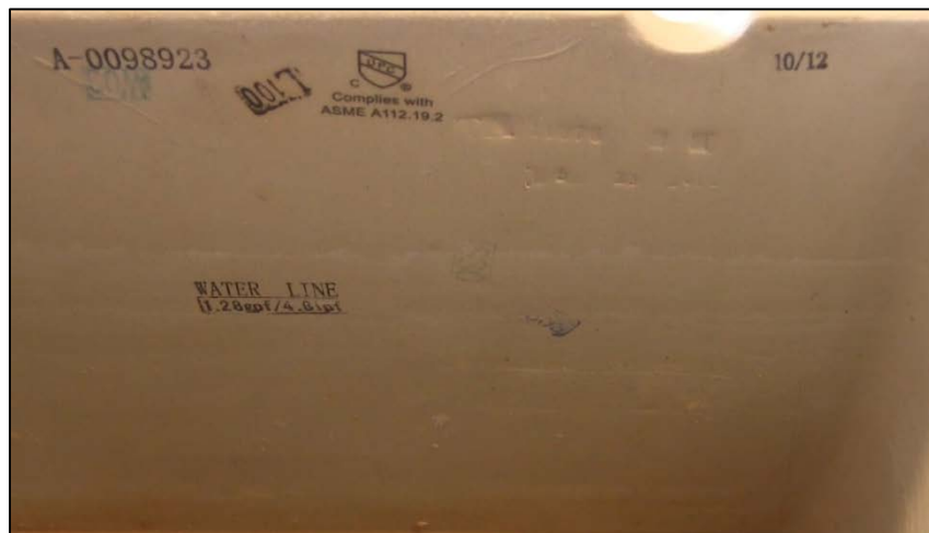
CAPTION 2. STAMPS FOUND INSIDE THE TOILET TANK INCLUDE MODEL NUMBER, AND HOW MUCH GALLONS PER FLUSH IS DISPENSED. WATER LINE INDICATES THE FILL LINE OF THE WATER WHEN SUPPLIED BACK TO THE TANK.
