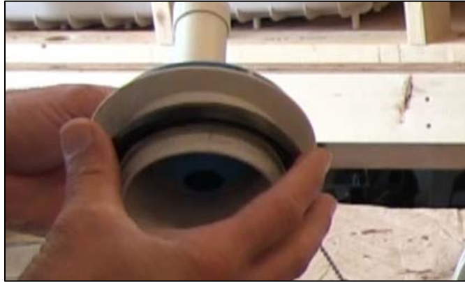
CAPTION 3. GASKET IS ATTACHED TO THE BOTTOM OF THE FLUSH VALVE.
