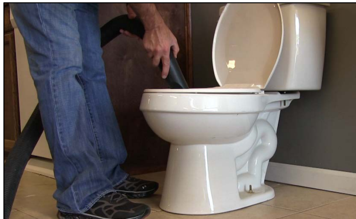
CAPTION 14. A SHOP VACUUM IS USED TO DRAIN THE WATER INSIDE THE TOILET BOWL.
