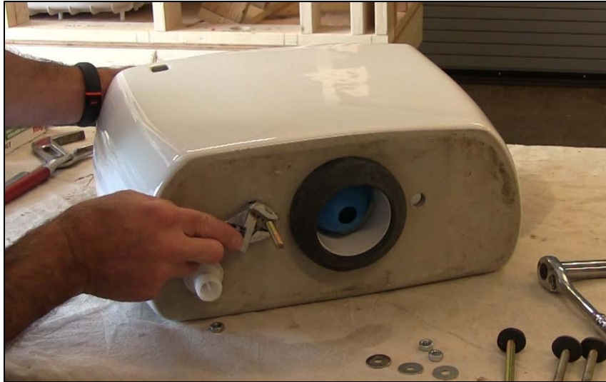
CAPTION 11. THE INSTRUCTOR TIGHTENS THE NUT AROUND THE BOLT USING A CRESCENT WRENCH.
