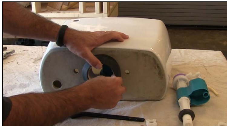
CAPTION 6. GASKET IS PLACED TO SEAL THE JOINT.
