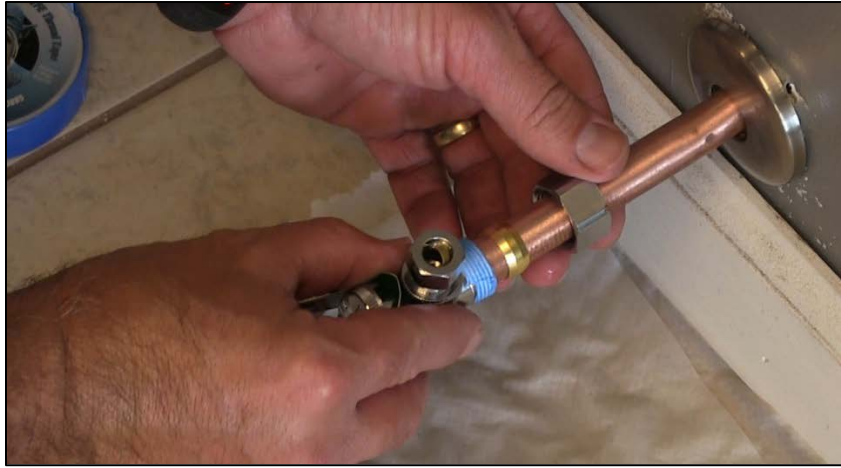
CAPTION 19. THE NUT, FERRULE, AND FITTING ARE PLACED ON THE PIPE.
