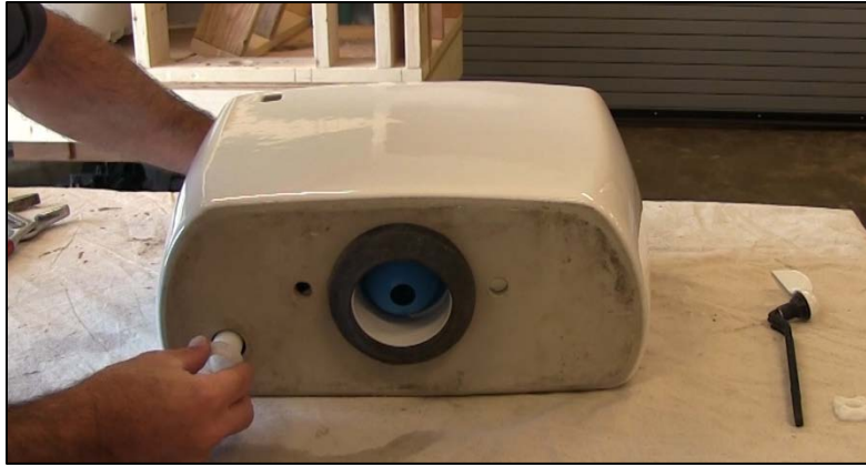
CAPTION 7. FILL VALVE IS INSTALLED ON THE TOILET TANK.
