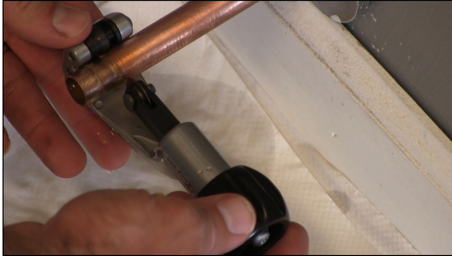
CAPTION 17. THE DENTED PART OF THE PIPE IS REMOVED.
