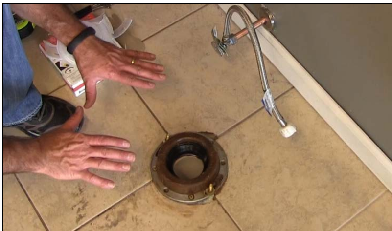
CAPTION 24. THE WAX RING IS SET ON THE FLANGE, WITH THE TWO BOLTS IN PLACE.
