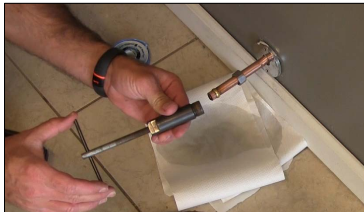
CAPTION 16. THE INSTRUCTOR IS READY TO REMOVE THE OLD FERRULE WITH A FERRULE REMOVING TOOL.
