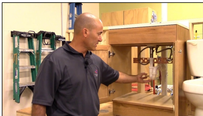
FIGURE 1. THE INSTRUCTOR STANDS IN FRONT OF A MOCK-UP SINK FIXTURE AND POINTS AT THE P-TRAP INSTALLED UNDERNEATH THE SINK
