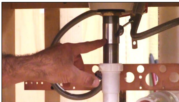
FIGURE 3. A CLOSE-UP PHOTO OF THE INSTRUCTOR POINTING AT THE TAILPIECE EXTENSION
