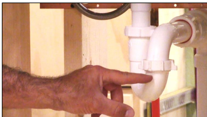
FIGURE 4. THE INSTRUCTOR POINTS AT THE P-TRAP. THE P-TRAP TRAPS WATER AND PREVENTS HARMFUL SEWER GASES FROM BACKING UP INTO THE HOME.
