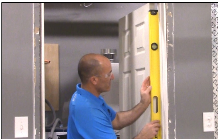
CAPTION 3. THE INSTRUCTOR CHECKS IF THE FRAMING IS PLUMB.
