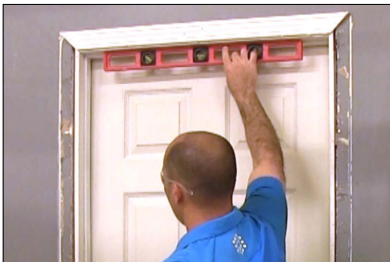
CAPTION 6. THE INSTRUCTOR CHECKS THE LEVEL OF THE TOP OF THE FRAME.
