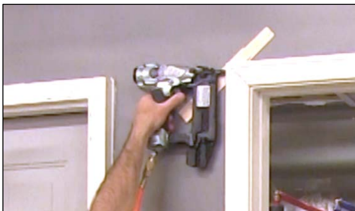
CAPTION 9. THE TOP AND SIDE CASING ARE FLUSH BY PLACING A SHIM BENEATH THE 45-DEGREE ANGLE ENDS OF THE CASINGS.
