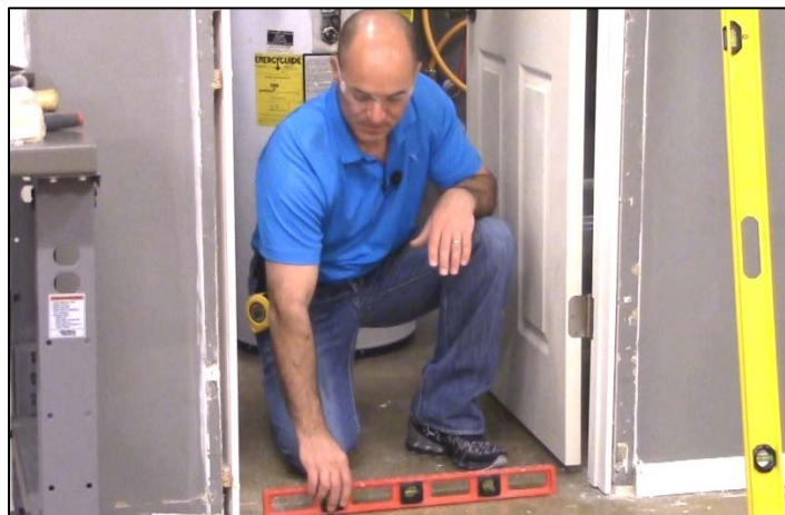
CAPTION 1. THE INSTRUCTOR CHECKS THE LEVEL OF THE FLOOR.
