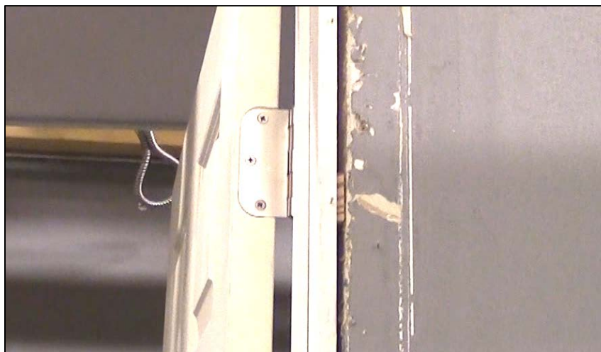
CAPTION 5. A SHIM IS PLACED IN THE GAP, RIGHT BEHIND ONE OF THE DOOR'S HINGES.
