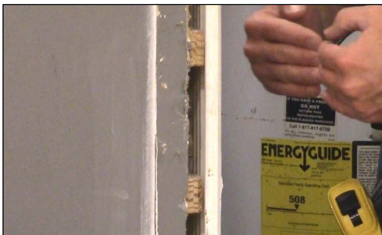
CAPTION 7. TWO SHIMS ARE PLACED BEHIND THE DOOR LATCH
