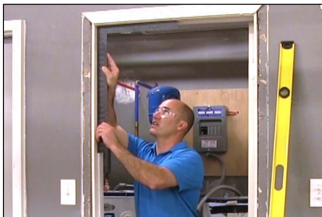
CAPTION 2. THE INSTRUCTOR USES A SPEED SQUARE TO CHECK THE DOOR OPENING CORNER.
