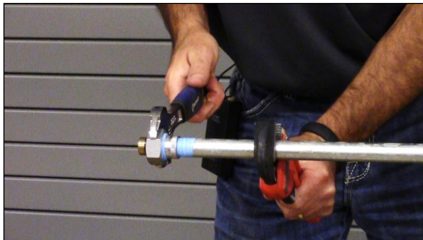
CAPTION 21. THE FITTING IS TIGHTENED USING A CRESCENT WRENCH.
