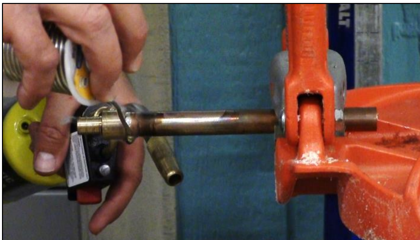
CAPTION 9. SOLDER IS APPLIED ON THE JOINT.
