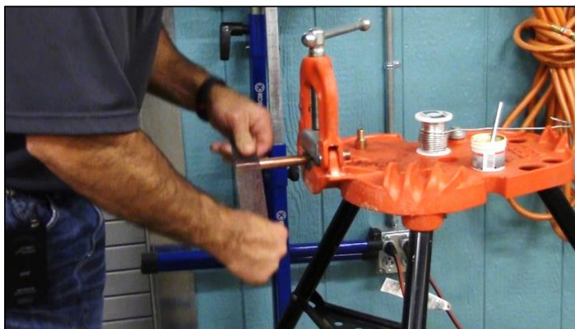
CAPTION 5. THE INSTRUCTOR CLEANS THE COPPER PIPE WITH AN EMERY CLOTH.
