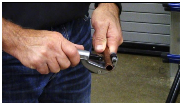
CAPTION 3. THE INSTRUCTOR DEMONSTRATES HOW TO CUT THE PIPE USING THE PIPE CUTTER.
