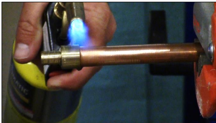
CAPTION 8. THE INSTRUCTOR HEATS THE PIPE WITH THE AUTO TORCH.
