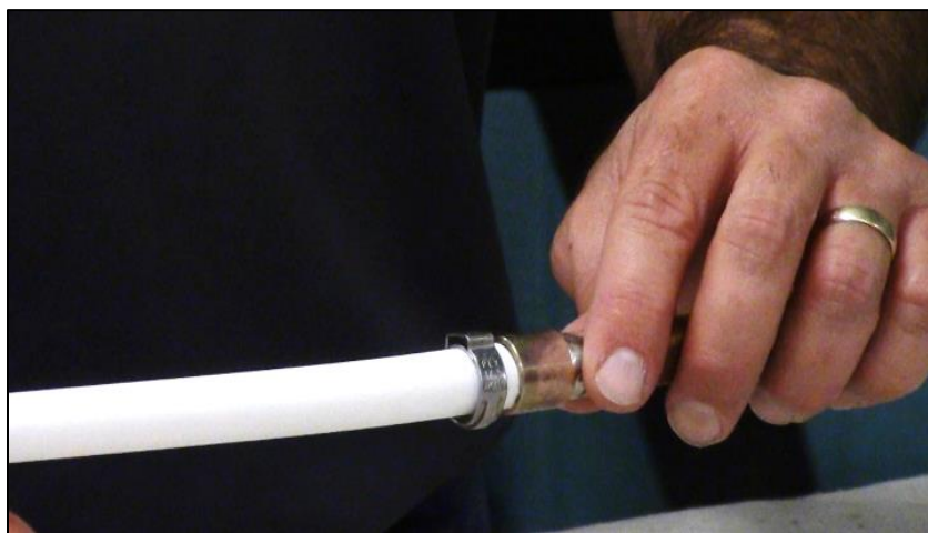
CAPTION 14. THE PINCH RING IS PLACED AN EIGHTH OF AN INCH AWAY FROM THE END OF THE PEX PIPE.
