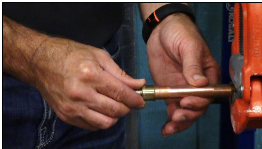
CAPTION 7. THE FITTING IS PLACED ON THE PIPE.
