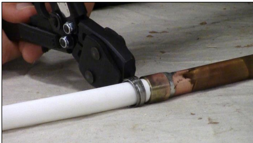
CAPTION 15. THE PINCH RING IS TIGHTENED AROUND THE PIPE USING A RATCHET TOOL.
