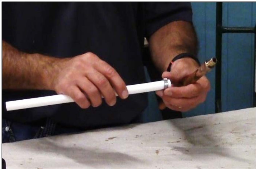
CAPTION 13. THE PINCH RING IS PLACED AROUND THE PEX PIPE
