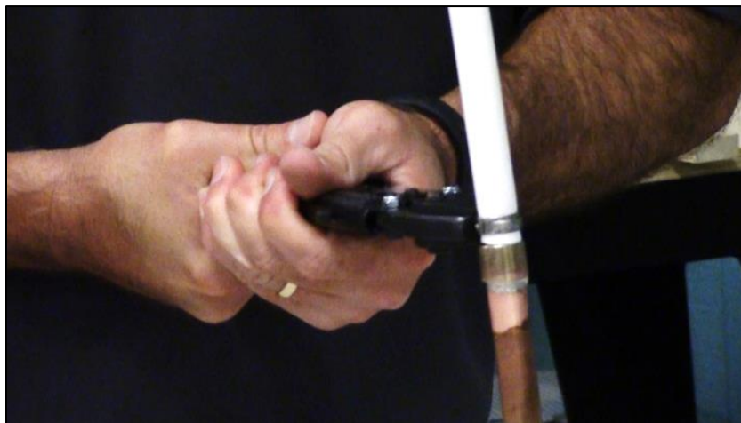
CAPTION 16. THE INSTRUCTOR TIGHTENS THE PINCH RING AROUND THE PEX PIPE.
