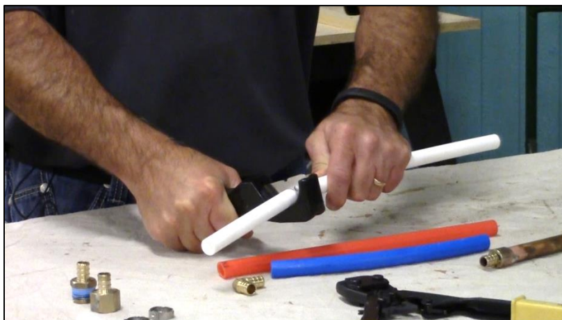
CAPTION 11. THE INSTRUCTOR DEMONSTRATES HOW TO CUT A PEX PIPE USING THE PEX PIPE CUTTER.
