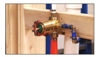
CAPTION 2 A CLOSE-UP PHOTO OF THE INSTALLED MIXING VALVE
