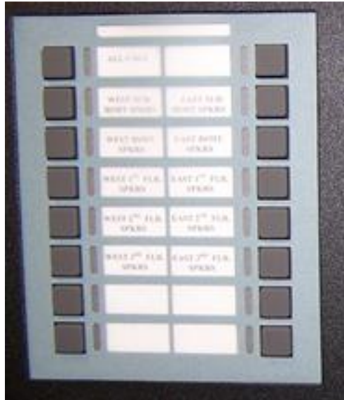
Fig. 15-5 Alarm panels were designed with discrete panels that lit or blinked with each alarm. Buttons were used to acknowledge each alarm point.
