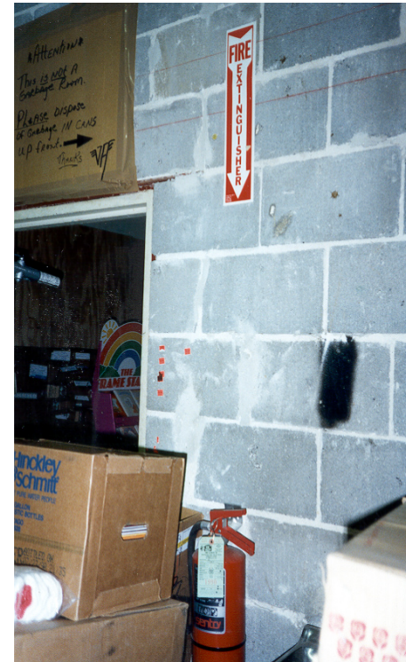
Blocked extinguisher
