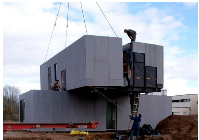
FIGURE 27 - MODULAR HOUSE UNDER CONSTRUCTION BY CG ARCHITECTS, CROSSBOX.
