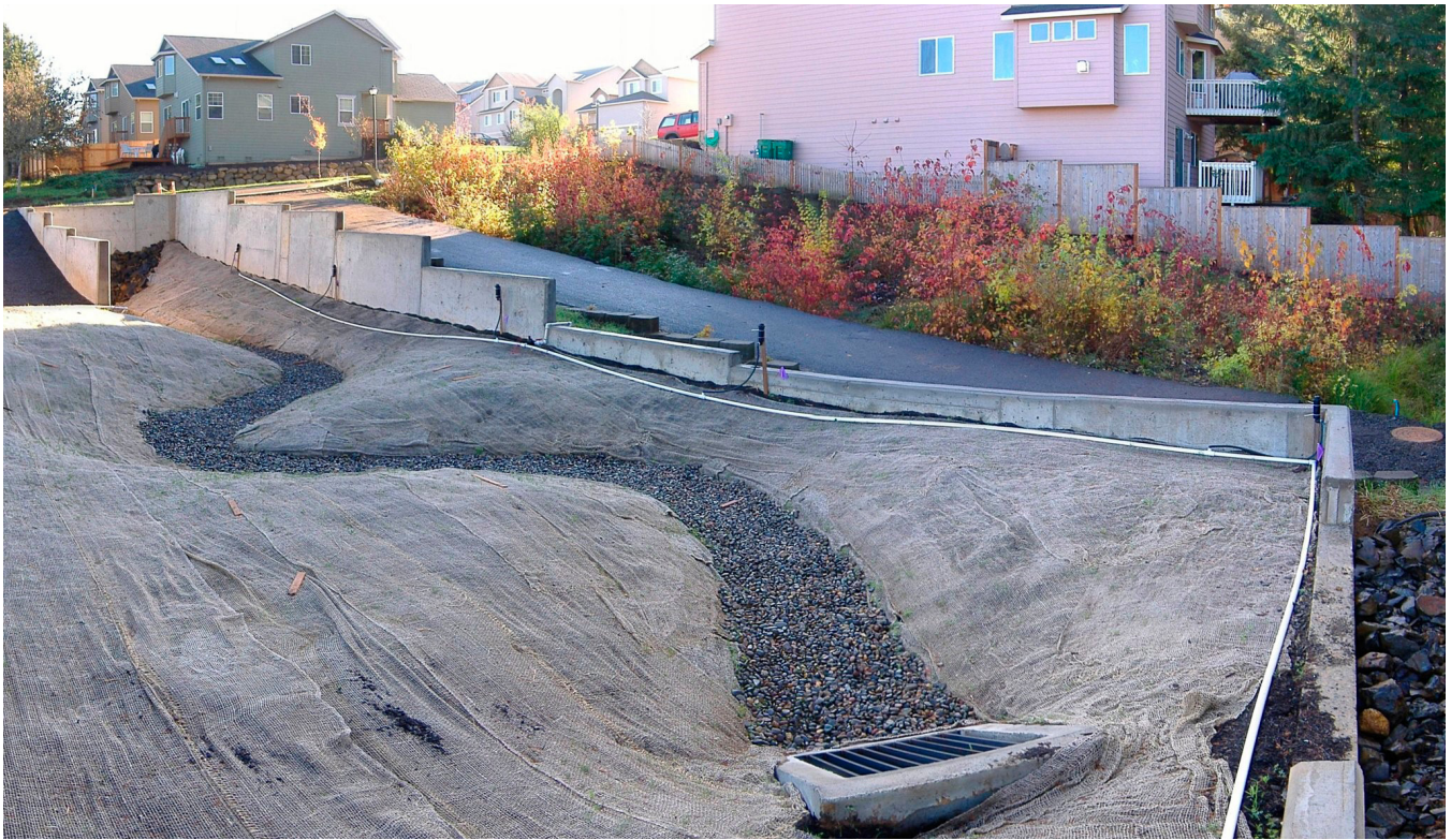
FIGURE 10 - URBAN BIOWALE UNDER CONSTRUCTION. THESE SYSTEMS HELP TO ABSORB AND TREAT STORMWATER RUNOFF FROM THE BUILT ENVIRONMENT AND CAN BE USED TO PROVIDE A BETTER URBAN SPACE.
