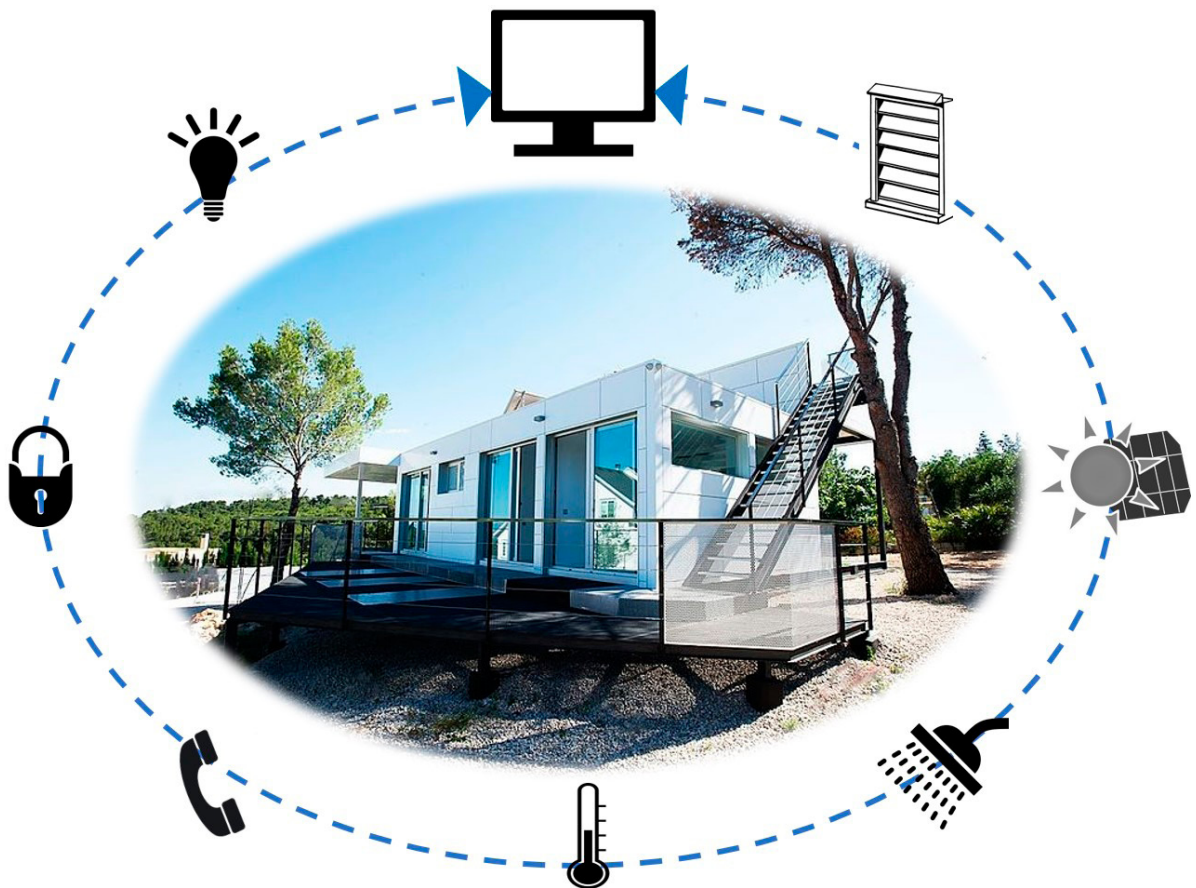
FIGURE 19 - MODULAR AND MANUFACTURED HOMES OFFER GREAT OPPORTUNITIES FOR BUILDING AUTOMATED SYSTEMS SINCE THEY CAN BE DESIGNED AND INSTALLED DURING THE MANUFACTURING PROCESS. THIS PICTURE IS A MODULAR HOME CONSISTING OF 6 PREFABRICATED MODULES IN VALENCIA, SPAIN.
