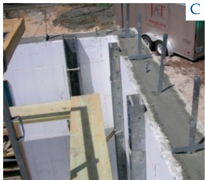
FIGURE 22 - (A) PREFABRICATED STRUCTURAL INSULATED PANELS, (B) AERATED AUTOCLAVED CONCRETE, AND (C) INSULATED CONCRETE FORMS.
