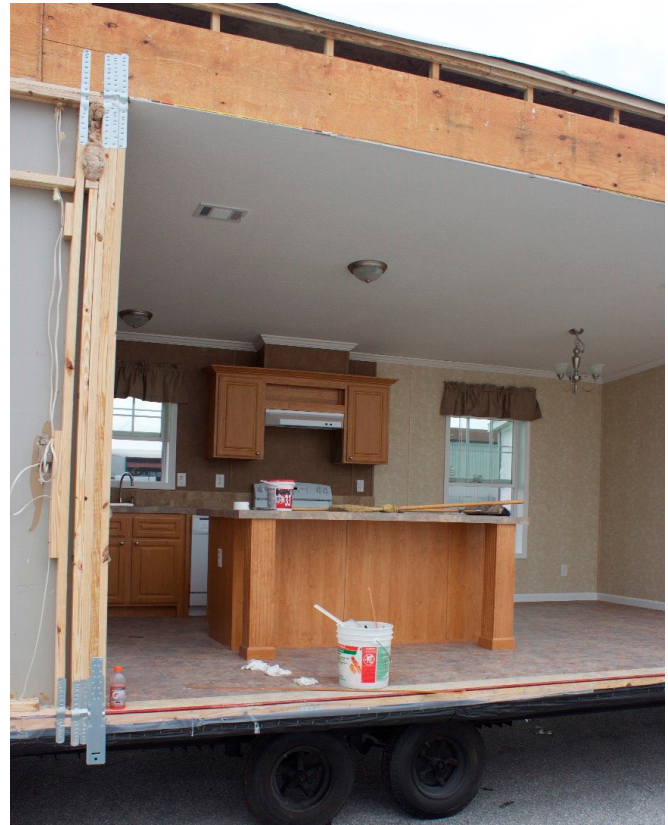
FIGURE 1.60 AND 1.61: TRIM WORK, REMAINING ELECTRICAL INSTALLMENT, AND OTHER FINISHES ARE DONE IN THIS STATION
