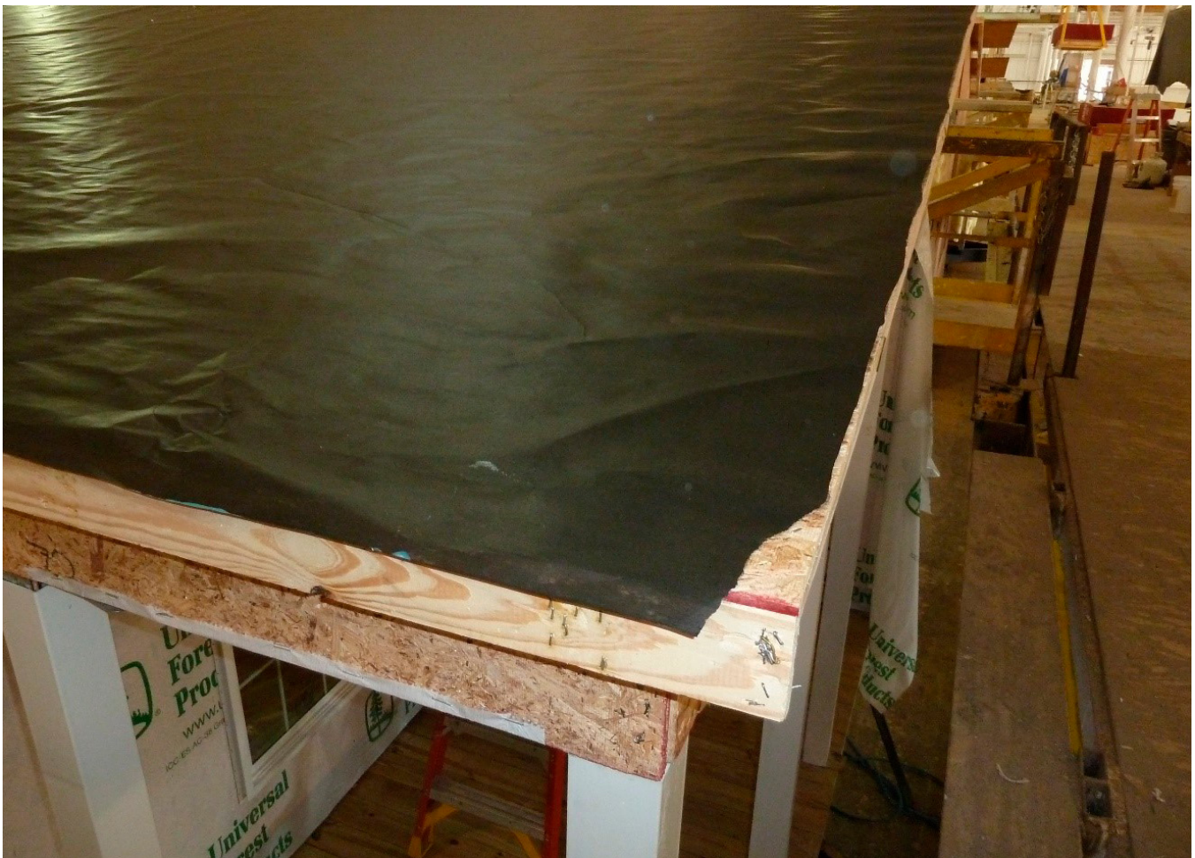
FIGURE 1.56: EXTERIOR SHEATHING BEING INSTALLED ON THE EXTERIOR OF THE HOME
