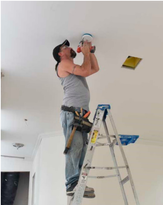
FIGURE 1.60 AND 1.61: TRIM WORK, REMAINING ELECTRICAL INSTALLMENT, AND OTHER FINISHES ARE DONE IN THIS STATION
