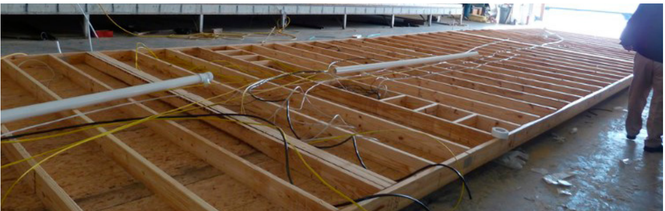
FIGURE 1.13: PLUMBING INSTALLATION WITHIN THE FLOOR-FRAMING STATION
