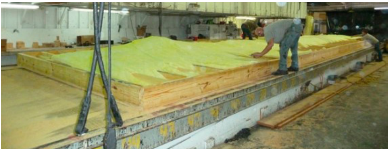
FIGURE 1.15 AND 1.16: INSULATION IS APPLIED ON THE WOODEN FLOORING
