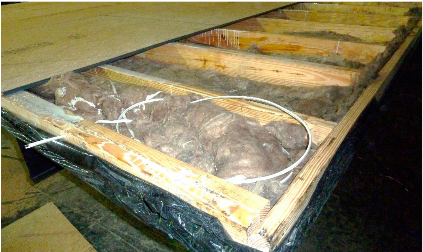
FIGURE 1.12: ELECTRICAL INSTALLATION IN THE FLOOR
