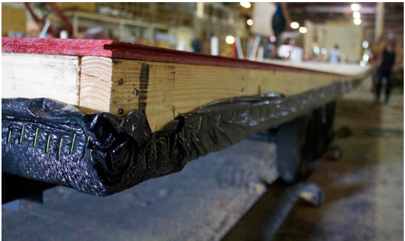
FIGURE 1.18, 1.19: THE CHASSIS IS MOVED AND TURNED OVER TO ALLOW FOR FRAMING.
