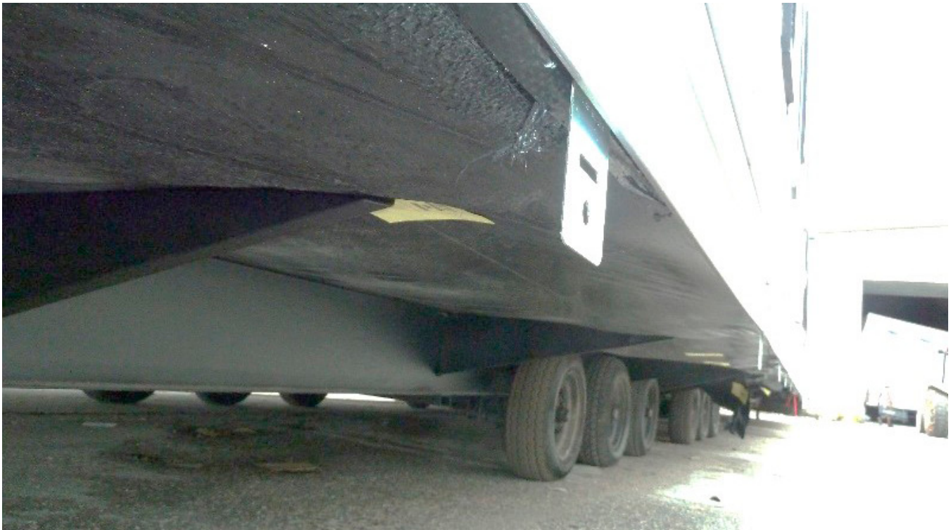
FIGURE 1.8: THE OUTRIGGER IS AN EXTENDED PIECE COMING OUT AND ATTACHED TO THE I-BEAM. IT EXTENDS TO CARRY ALL THE LOAD TO THE EDGE OF THE UNIT.
