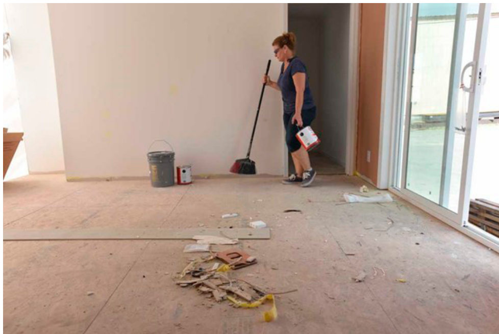
FIGURE 1.64: FINAL CLEANING OF THE UNIT
