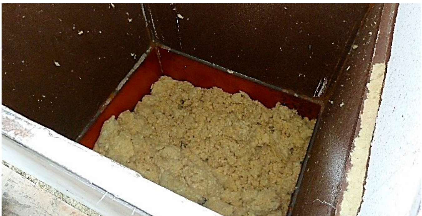
FIGURE 1.47: THE INSULATION IS BLOWN INTO THE VOID BETWEEN THE TRUSSES.
