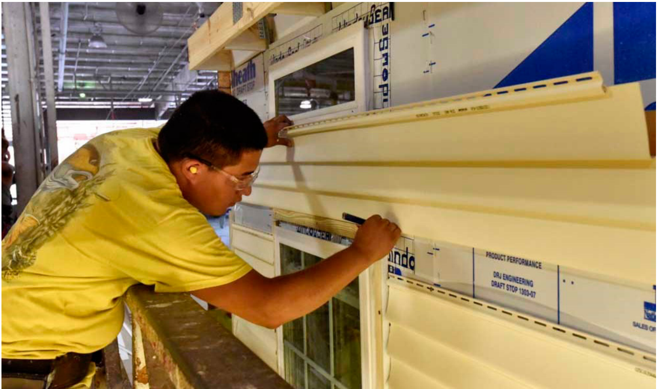
1.56: EXTERIOR SHEATHING BEING INSTALLED ON THE EXTERIOR OF THE HOME
