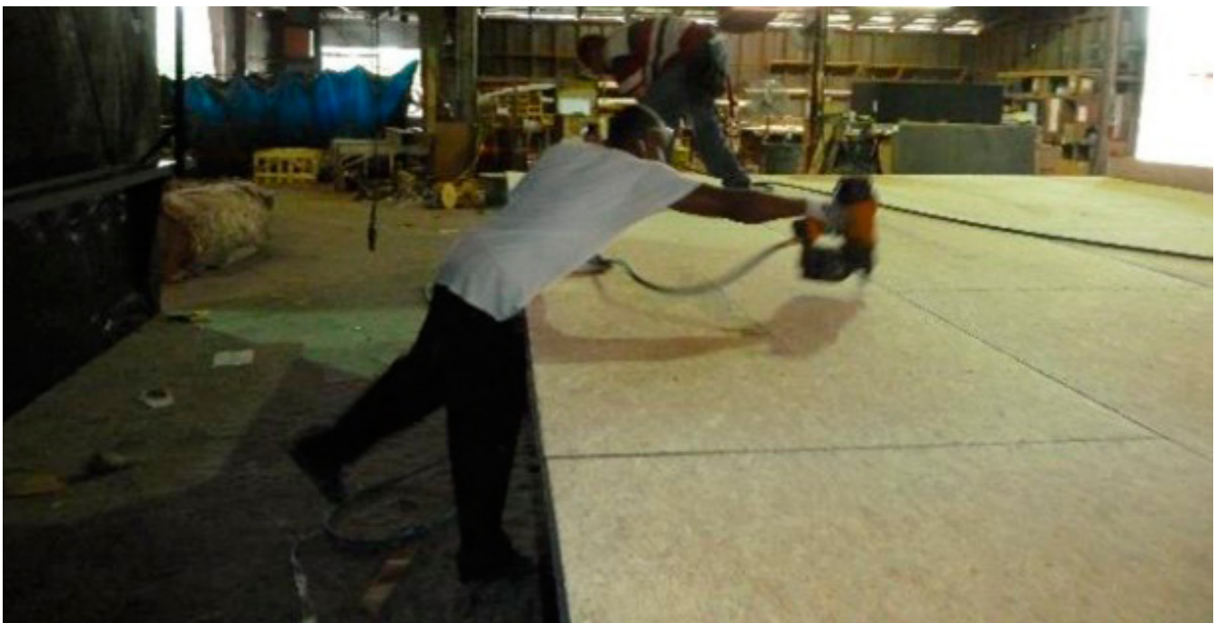
FIGURE 1.21: THE FLOOR DECK INSTALLATION
