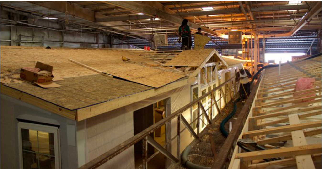
FIGURE 1.50: SHEATHING BEING APPLIED TO THE ROOF.
