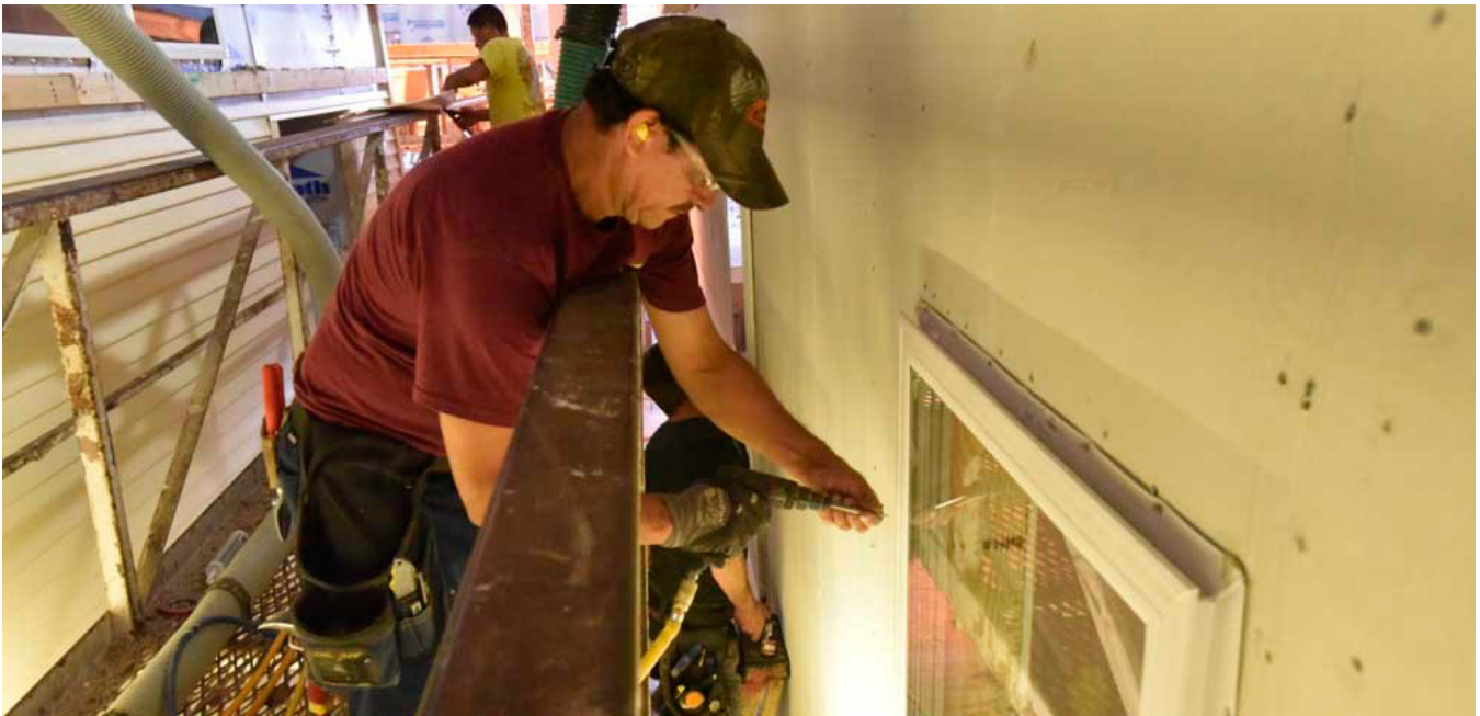
FIGURE 1.54: WINDOWS ARE SET AND FASTENED.
