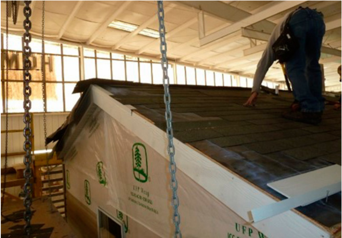
FIGURE 1.57: SHINGLES ARE BEING LAID AND NAILED TO THE ROOF.
