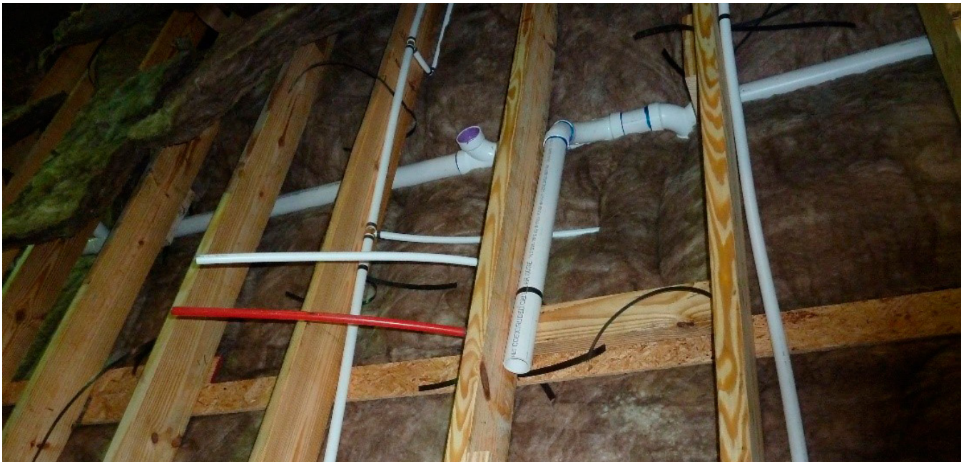
FIGURE 1.14: PLUMBING INSTALLATION WITHIN THE FLOOR-FRAMING STATION
