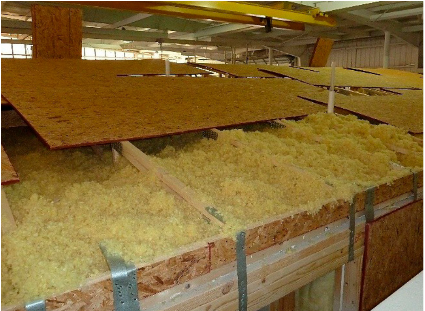
FIGURE 1.48, AND 1.49: THE INSULATION IS BLOWN INTO THE VOID BETWEEN THE TRUSSES.
