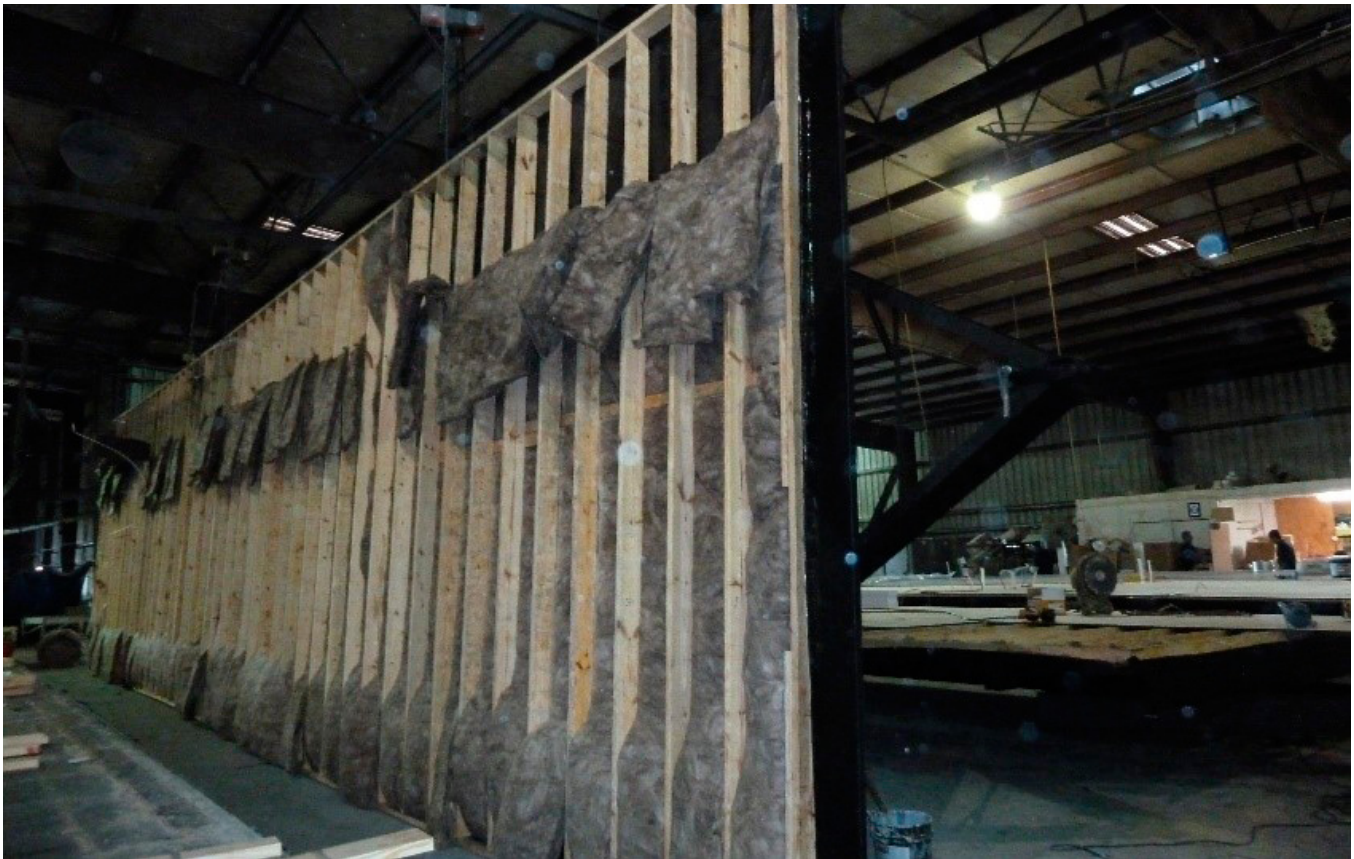
FIGURE 1.20: THE CHASSIS IS MOVED AND TURNED OVER TO ALLOW FOR FRAMING.
