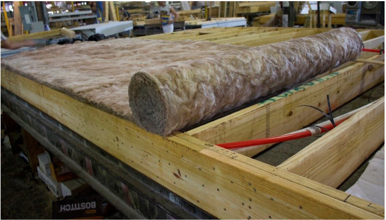
FIGURE 1.16: INSULATION IS APPLIED ON THE WOODEN FLOORING
