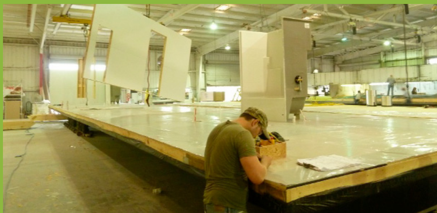
FIGURE 3.3: FLOORING IS ALMOST READY IN THE FLOORING STATION
