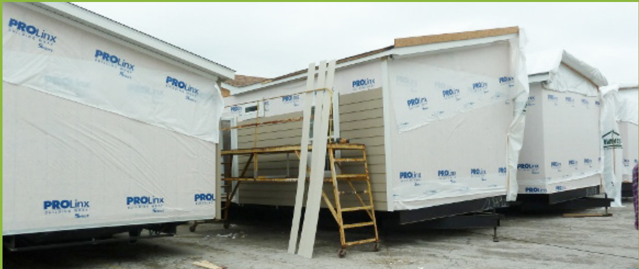
FIGURE 1.9: HUD-CODE UNIT ON A CHASSIS
