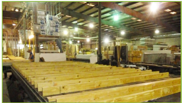
FIGURE 2.5: JIGS ARE USED TO BUILD LEVELED, SQUARED AND PRECISE FLOORS AND WALLS
