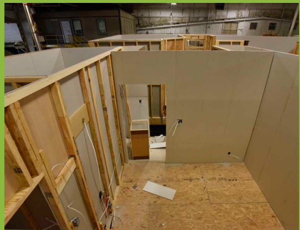
FIGURE 3.5: INTERIOR WALLS ARE BUILT IN THE WALL ASSEMBLY STATION
