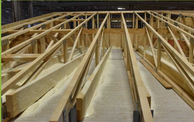
FIGURE 3.6: TRUSSES BEING ASSEMBLED ON THE ROOFING STATION
