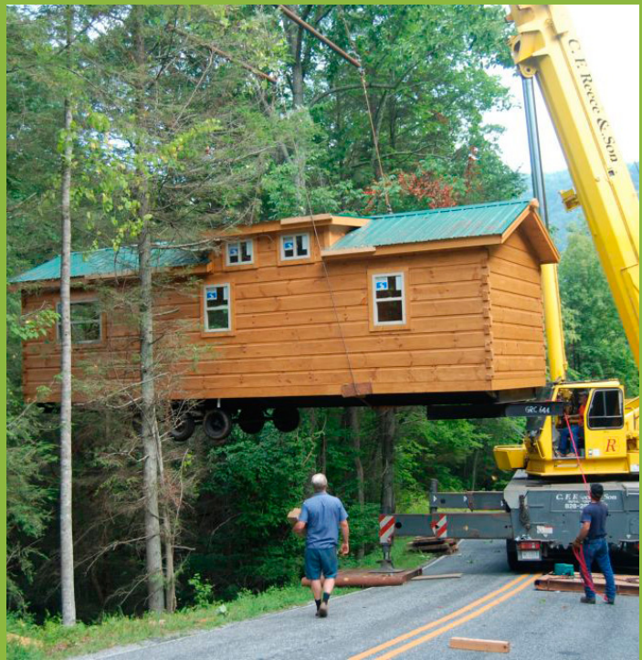
FIGURE 1.19: PARK MODEL BEING MOVED WITH A CRANE DURING INSTALLATION
