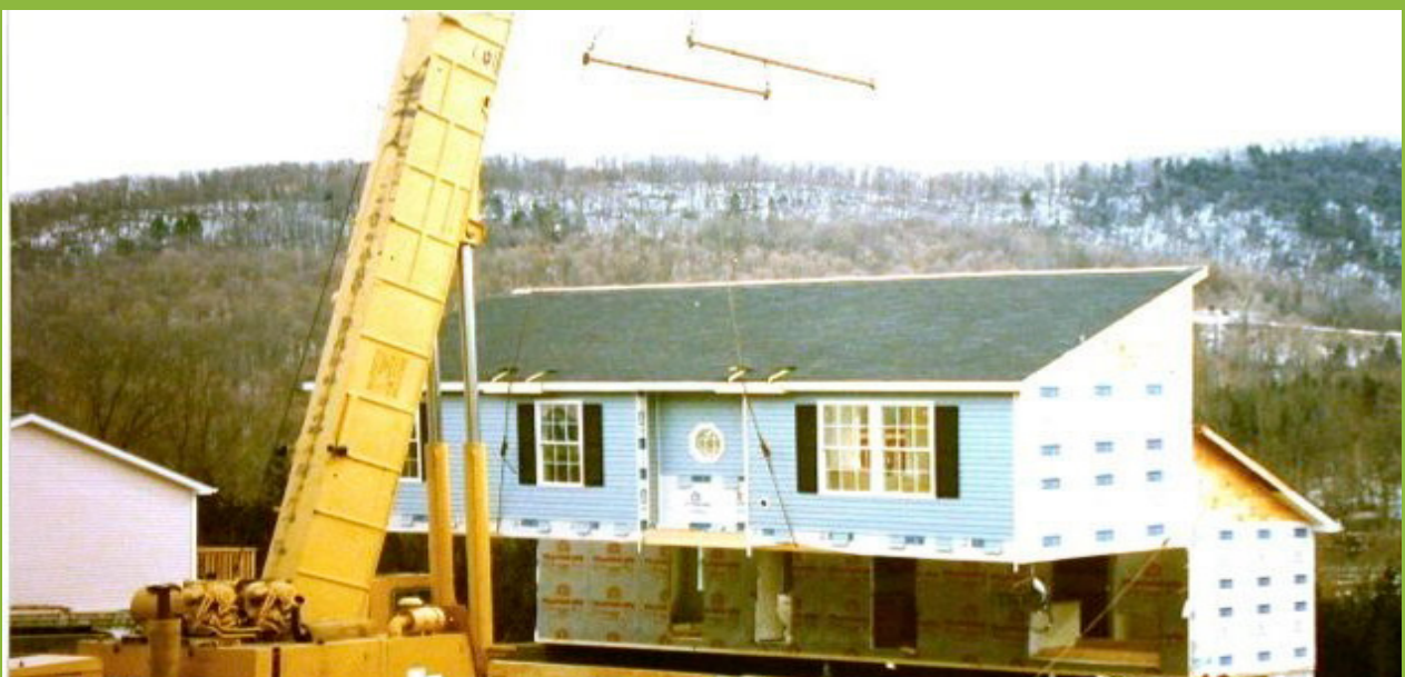
FIGURE 1.16: MODULAR HOME UNIT BEING ERECTED ON SITE USING CRANES
