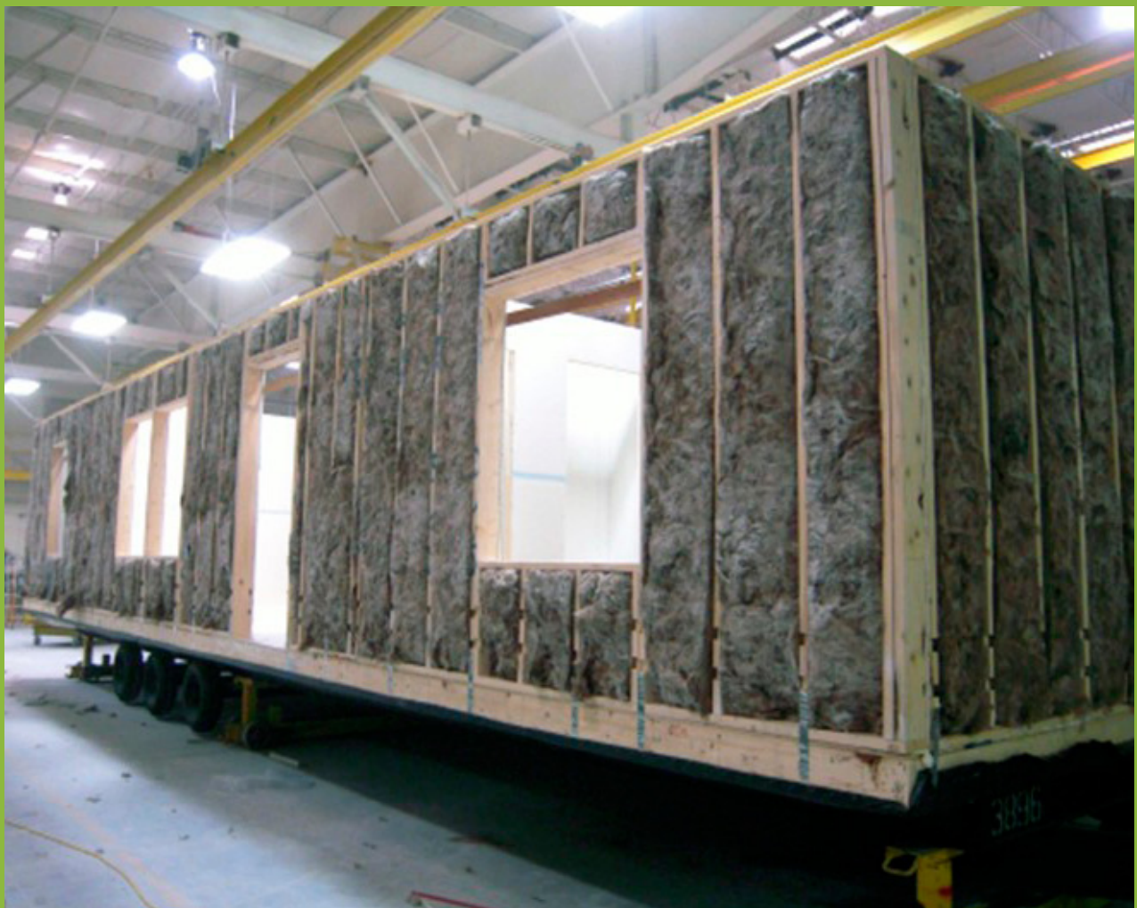
FIGURE 1.8: THE MANUFACTURED HOME IS BUILT FROM INSIDE TO OUTSIDE
