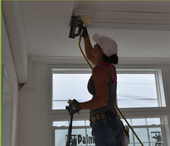
FIGURE 3.8: TRIM-WORK AND FINAL FINISHING IN THE INTERIOR OF THE UNIT
