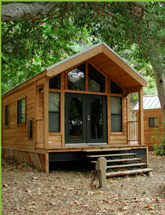
FIGURE 1.18: PARK MODEL INSTALLED
