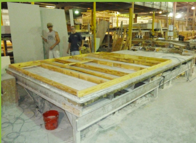
FIGURE 3.4: WALLS BEING COMPLETED IN THE OFFLINE WALL STATIONS
