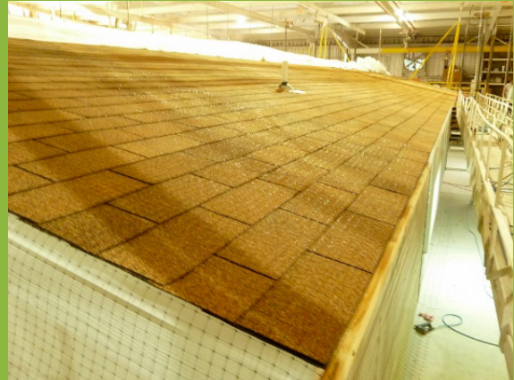
FIGURE 3.7: SHINGLES ARE READY IN THE ASSEMBLY ROOFING STATION
