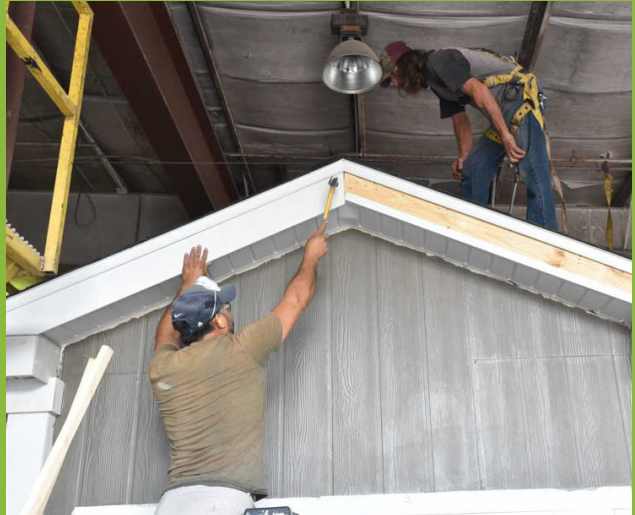
FIGURE 3.9: SOFFITS AND TRIM-WORK ON THE EXTERIOR OF THE UNIT BEING INSTALLED
