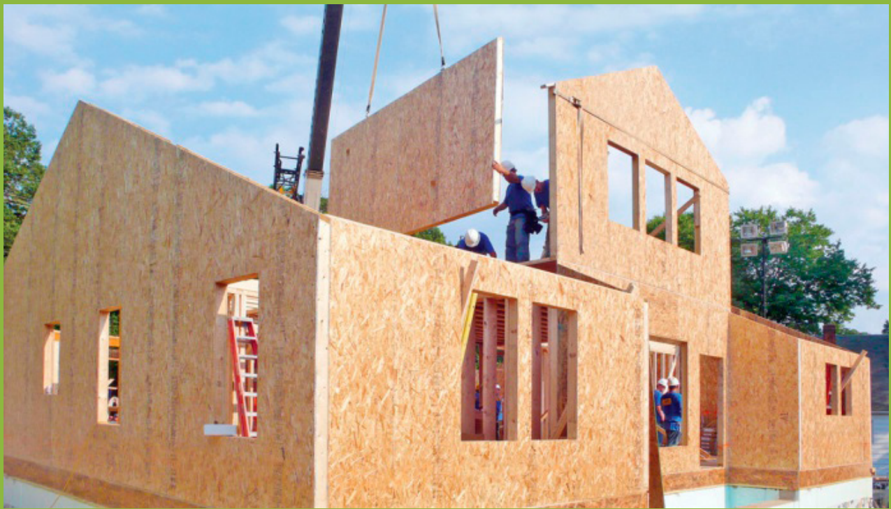
FIG. 1.22: STRUCTURAL INSULATED PANELS BEING ASSEMBLED INTO A BUILDING
