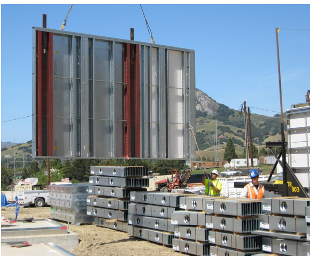
FIGURE 3.15 - THE STEEL PREFABRICATED PANEL READY TO BE INSTALLED. (SOURCE: KH&S INTERNATIONAL)
