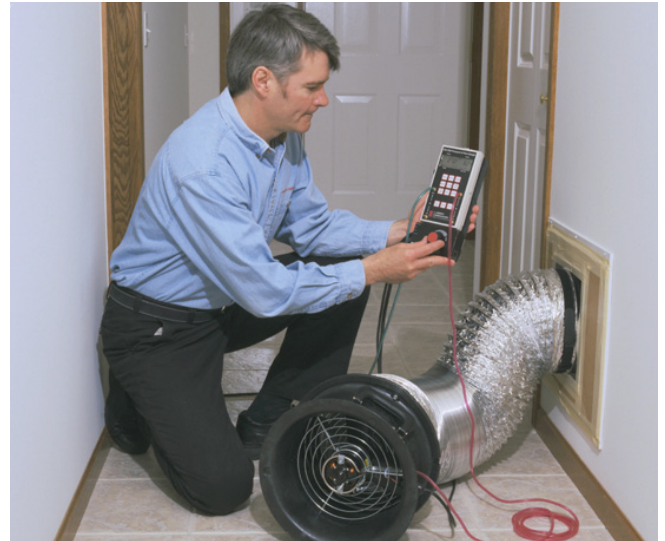
FIGURE 2.36 - FOR TESTING DUCT SYSTEM AIR LEAKAGE, A FAN IS DIRECTLY CONNECTED TO HVAC SYSTEM TO PRODUCE AIR PRESSURE. (SOURCE: KELLY HEATING AND AIR CONDITIONING)
