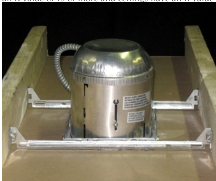
FIGURE 1.10 - A PROPERLY INSTALLED IC-RATED RECESSED OR 'CAN' LIGHT WHICH CAN BE SAFELY COVERED WITH INSULATION.
