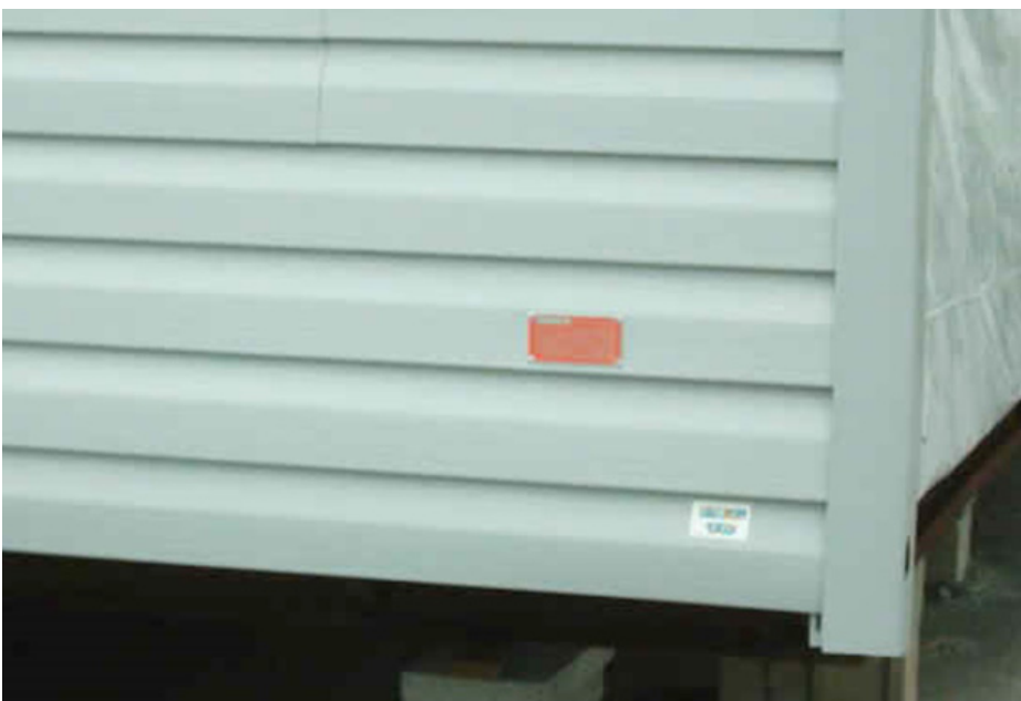
FIGURE 1.5 THE CERTIFICATION LABEL MUST BE PERMANENTLY ATTACHED TO EVERY MANUFACTURED HOME SOLD IN THE U.S.
