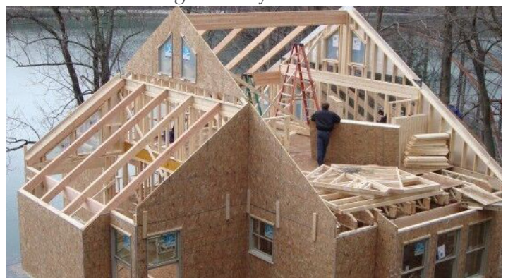
FIGURE 3.1 INSTALLATION OF A PANELIZED WOODEN WALL. (SOURCE: LOGANGATE TIMBER HOMES)
