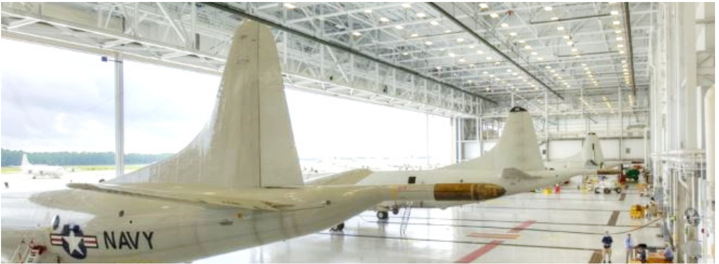
FIGURE 3.28 - JACKSONVILLE NAVAL AIR STATION P302V MAINTENANCE HANGAR. TO MEET THE U.S. NAVY'S DEMAND FOR MULTIPLE OPENINGS FOR VARIOUS AIRCRAFT, CLEAR SPANS OF 455 FEET AND 428 FEET WERE NECESSARY AT THE FRONT OF THE HANGAR. TO ACHIEVE THESE RECORD-SETTING CLEAR SPANS, HEAVY STRUCTURES DESIGNED THE HANGAR UTILIZING THREE-STORY-TALL BOX TRUSSES. DURING ERECTION, THESE ROBUST TRUSSES WERE ASSEMBLED IN SECTIONS ON THE GROUND, THEN LIFTED INTO PLACE WITH THE ENTIRE SYSTEM BEARING ON TEMPORARY SHORING TOWERS. THE STRUCTURE ALSO SUPPORTS MULTIPLE OVERHEAD CRANES FOR MAINTENANCE OF THE AIRCRAFTS. THE 3-D STRUCTURAL DESIGN PROVED TO BE OVER 25% MORE EFFICIENT THAN THE NEAREST CONVENTIONAL SOLUTION. THE SIZE, COMPLEXITY AND ECONOMY OF THIS SUCCESSFUL PROJECT DEMONSTRATES THE CAPABILITIES AND ADVANTAGES HEAVY STRUCTURES HAS TO OFFER. (SOURCE: BUTLER MANUFACTURING)
