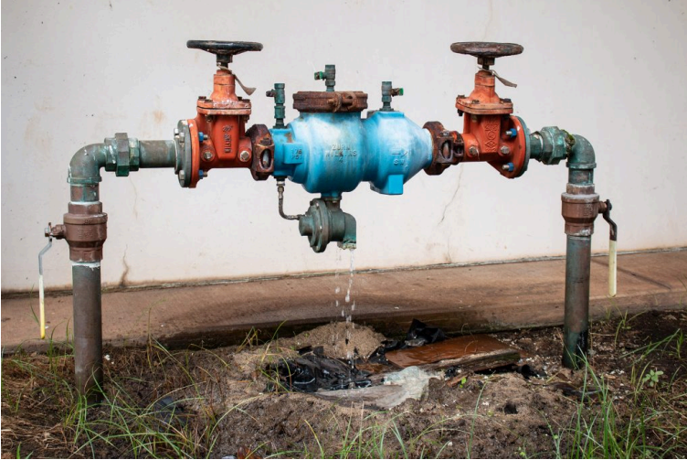
Reduced Pressure Zone Backflow Preventer by Gwen Arkin is licensed under CC BY 4.0
