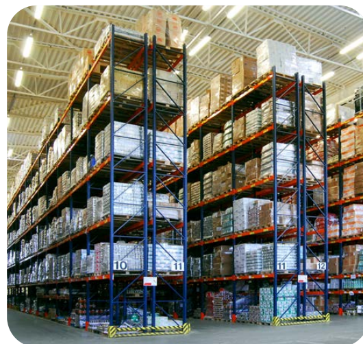
Figure 42. Double deep pallet racking. By Cortes003 (Own work) [CC BY-SA 3.0], via Wikimedia Commons.
