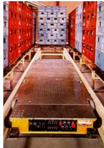
Figure 47. Unit load ASRS. Developed by LINCIS in Supply Chain Management Consortium.
