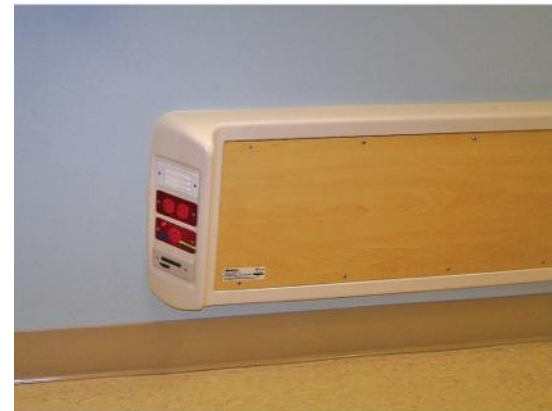
(B) RECEPTACLES BEHIND BED
