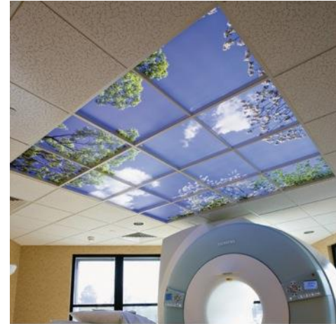
LUMINOUS SKYCEILING WITH RFI-FREE LED LIGHTING OVER MRI MACHINE
