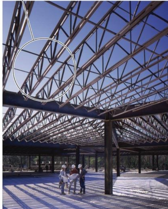
TYPICAL OPEN-WEB STEEL JOIST
