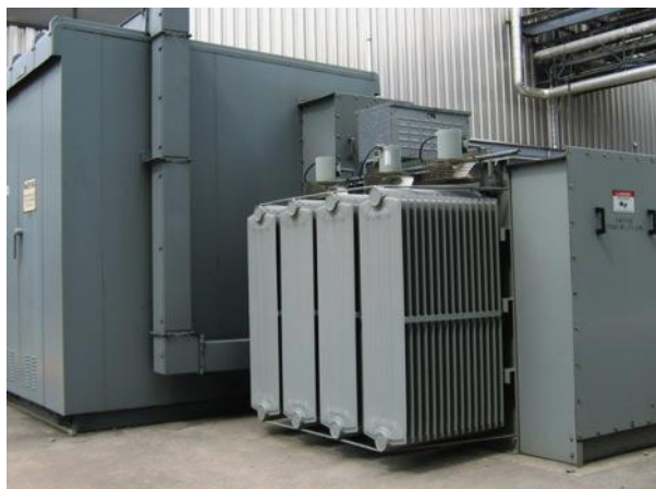
(A) DISTRIBUTION SWITCHGEAR
