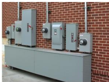
(B) COMMERCIAL ELECTRICAL SERVICE
