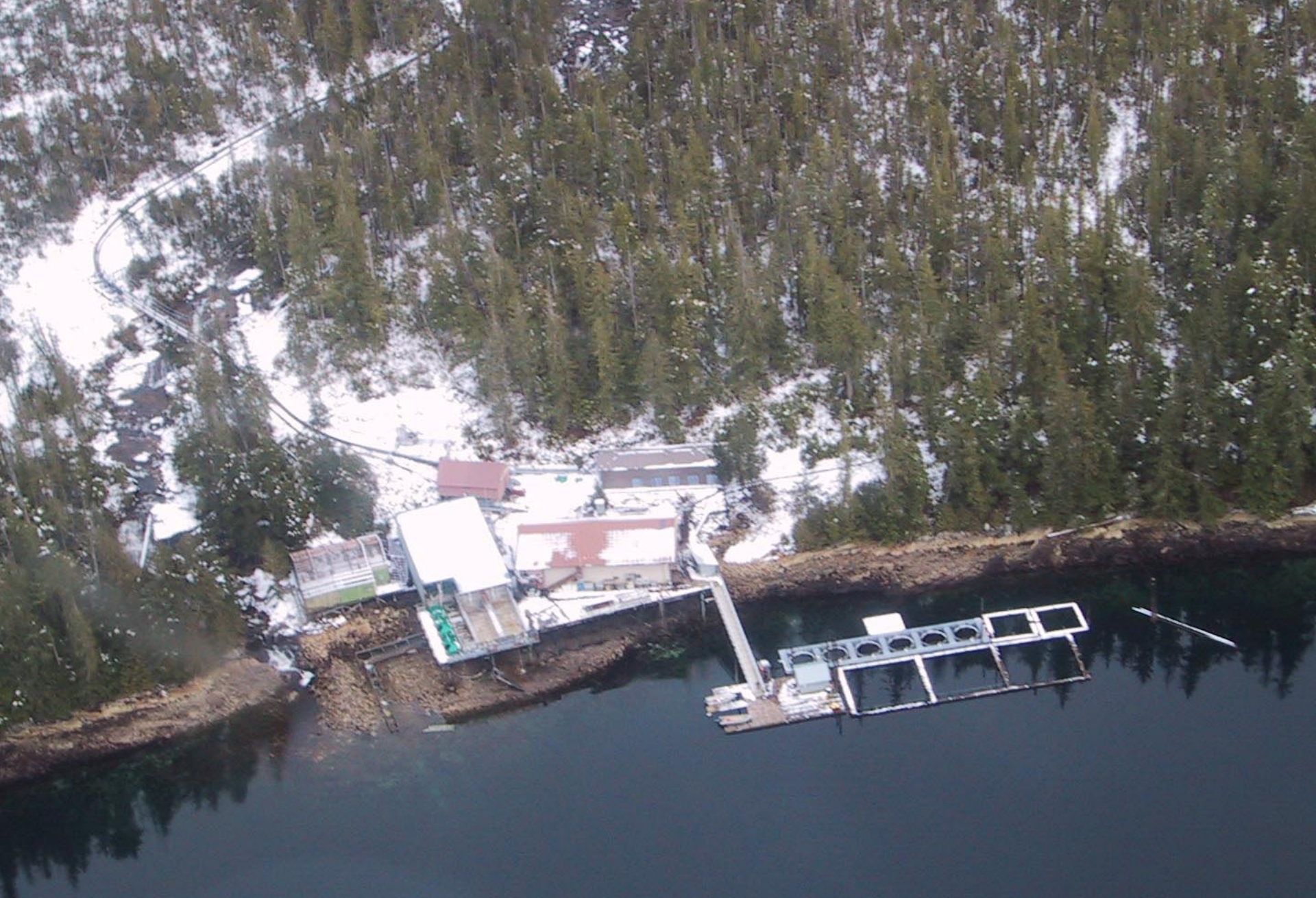
Burnett Inlet Hatchery
