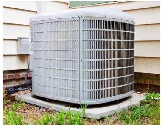
Central AC Condensing Unit
