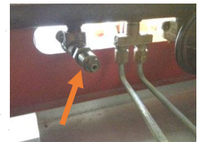
Manometer Connection Point at the burner orifice on an open burner range
