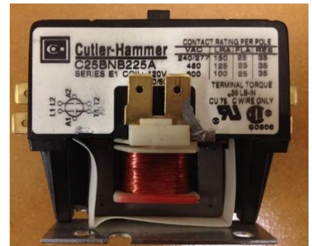
Contactor on Conveyor Oven
