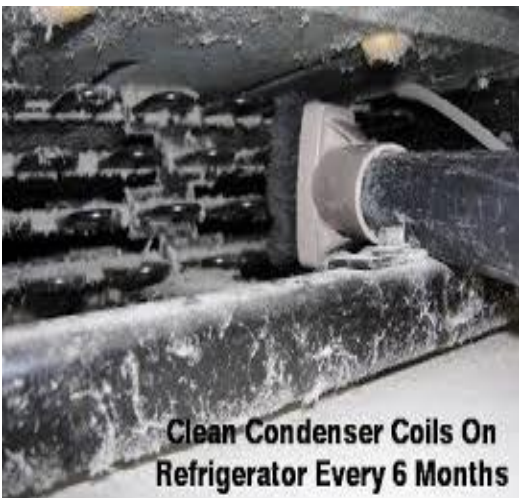
Cleaning a refrigerator condenser
