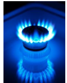
Natural Gas Burner
