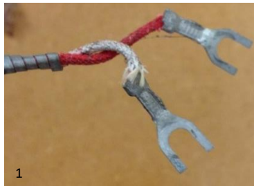
Thermopile gas valve electrical connections
