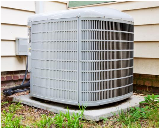
Central AC Condensing Unit
