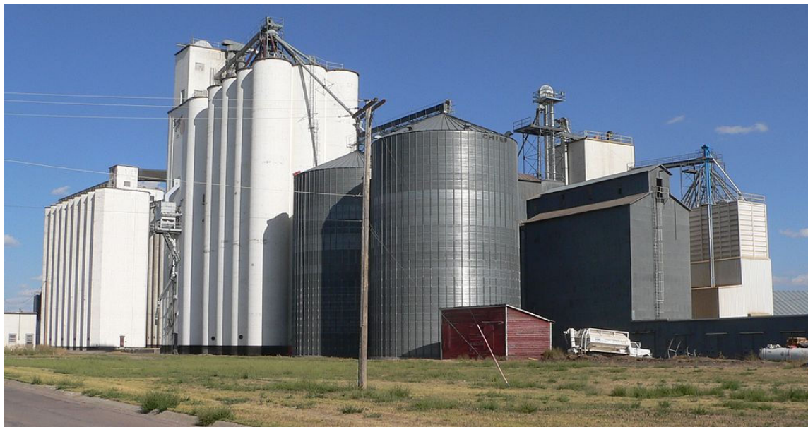
Figure 1-11: Grain elevators on a farm in Gordon, Nebraska. (Source: Ammodramus/Creative Commons (Public Domain)/ https://commons.wikimedia.org/wiki/File:Gordon,_Nebraska_grain_elevators_1.JPG )
