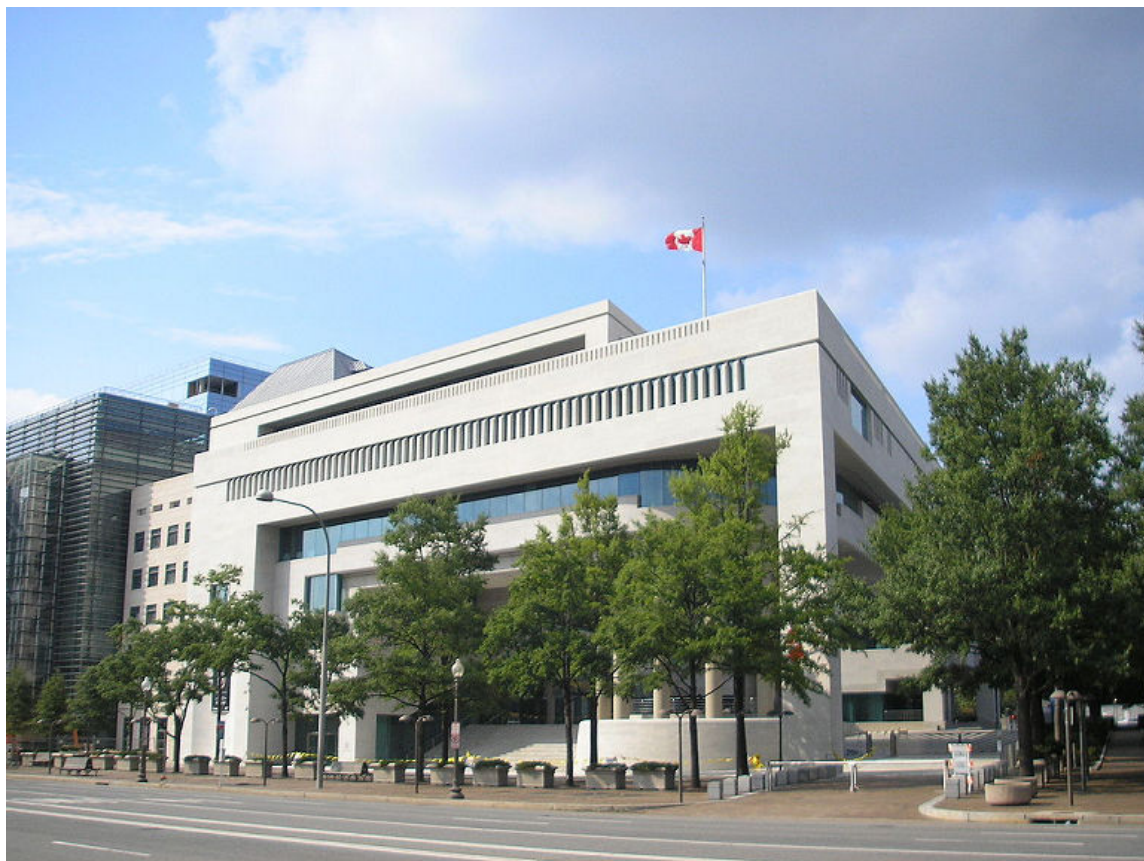
Figure 8–5: Large concrete planters act as a vehicle barrier to passing traffic in front of the Canadian Embassy in Washington, D.C. (Source: Gryffindor/Creative Commons (Public Domain)/ https://commons.wikimedia.org/wiki/File:Canadian_Embassy_DC_2007_002.jpg )
