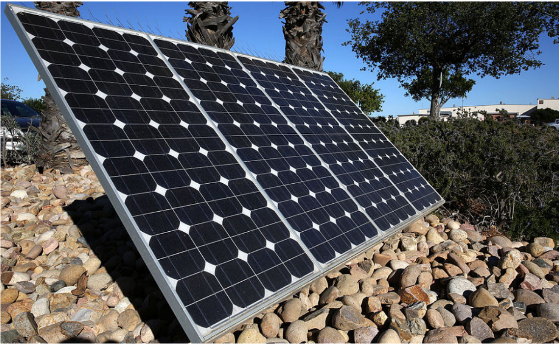
Figure 2-9: A solar panel on the grounds of the Marine Corps Air Station in Miramar, California is part of a microgrid providing warm water to the barracks and supporting backup power for a nearby landfill. (Source: Lance Cpl. Christopher Johns for the United States Marine Corps/Creative Commons (Public Domain)/ https://commons.wikimedia.org/wiki/File:Energy_assurance_only_a_microgrid_away_140113-M-OB827-007.jpg )
