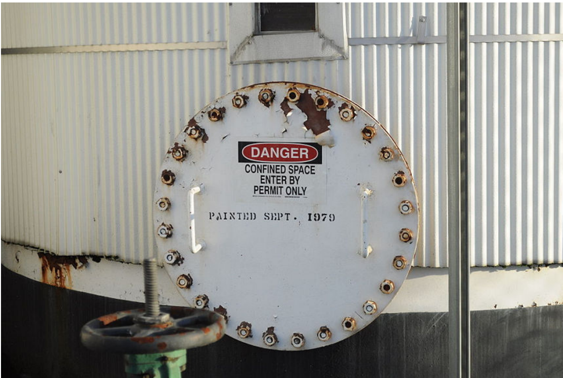
Figure 7-3: A notice warning about a confined space is posted on a piece of equipment. (Source: Joe Mabel/Creative Commons (CC BY-SA 3.0)/ https://commons.wikimedia.org/wiki/File:Confined_space_warning_01.jpg )
