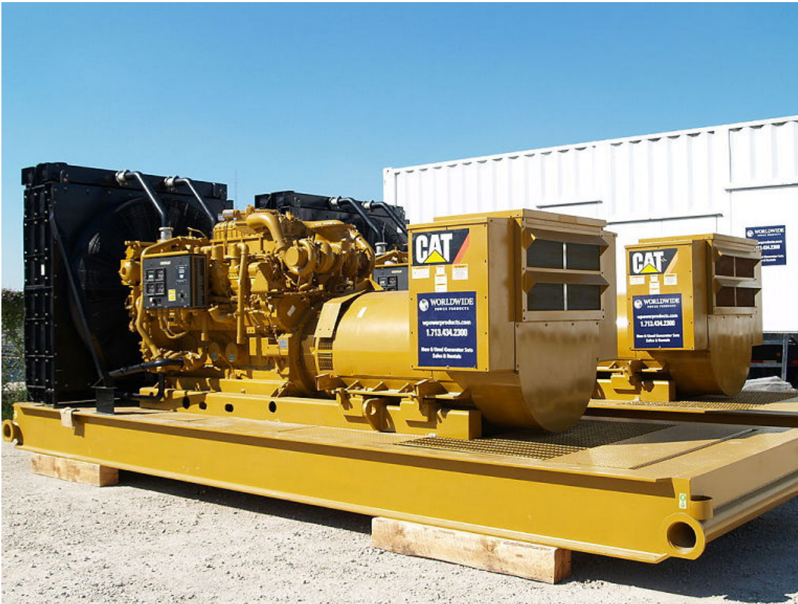
Figure 3-16: Any generator sets onsite, whether backup or primary, should be exercised on a monthly basis. (Source: StcudorPrewoP/Creative Commons (CC BY-SA 3.0)/ https://commons.wikimedia.org/wiki/File:Caterpillar_3512C_Generator_Set.JPG )
