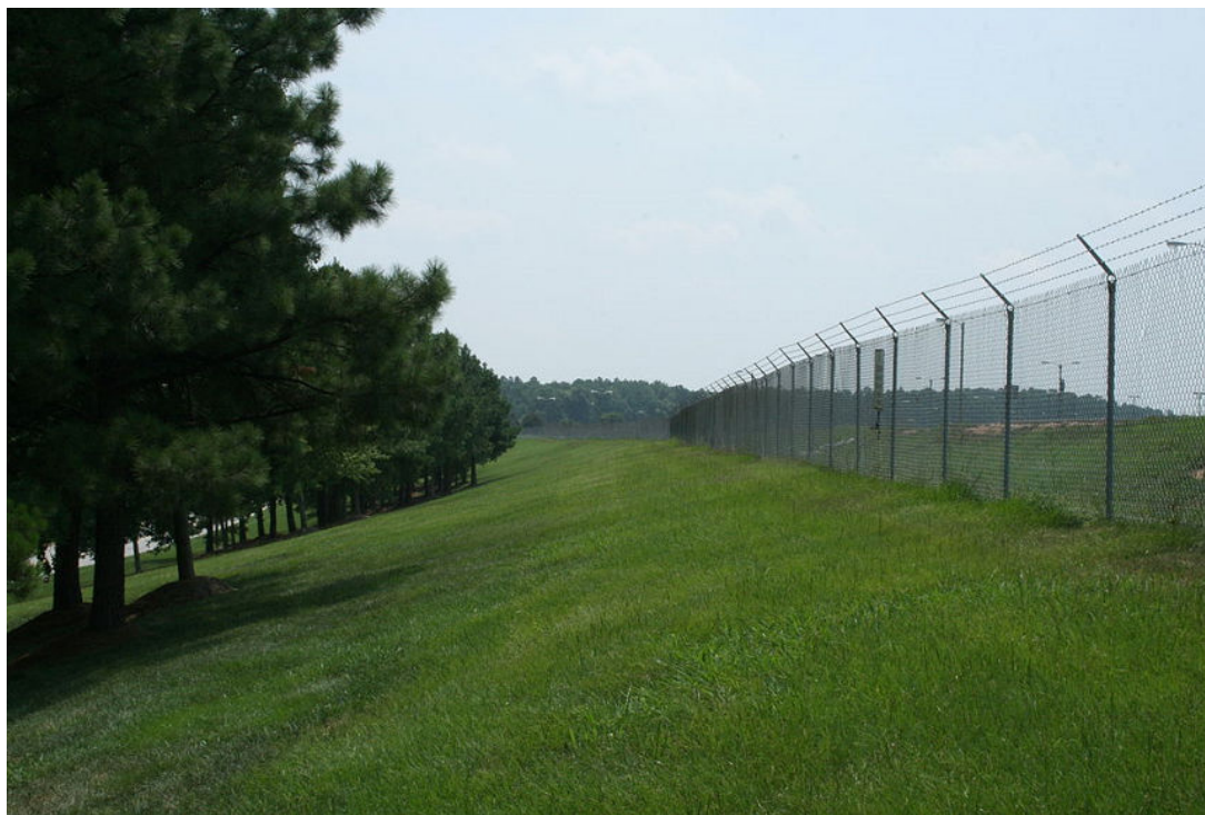
Figure 8-2: Fencing with the addition of barbed wire deters entry on to the property surrounding Raleigh-Durham International Airport. (Source: Ildar Sagdejev/Creative Commons (CC BY 3.0)/ https://commons.wikimedia.org/wiki/File:2008-07-30_Fence_along_Commerce_Blvd_at_RDU.jpg )
