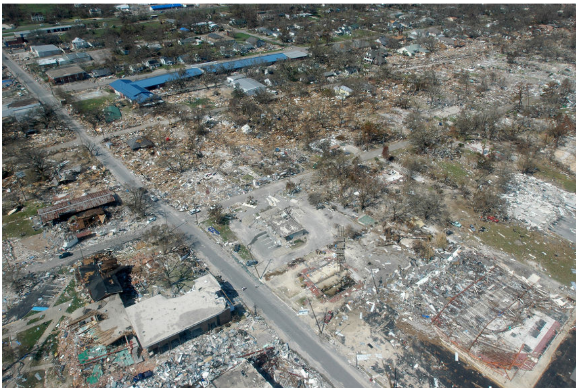
Figure 1-1: A hurricane—as evidenced by the damage seen here caused by Hurricane Katrina—can be a potential threat to MCO facilities. (Source: Federal Emergency Management Agency/Creative Commons (Public Domain)/ https://commons.wikimedia.org/wiki/File:Hurricane_katrina_damage_gulfport_mississippi.jpg )
