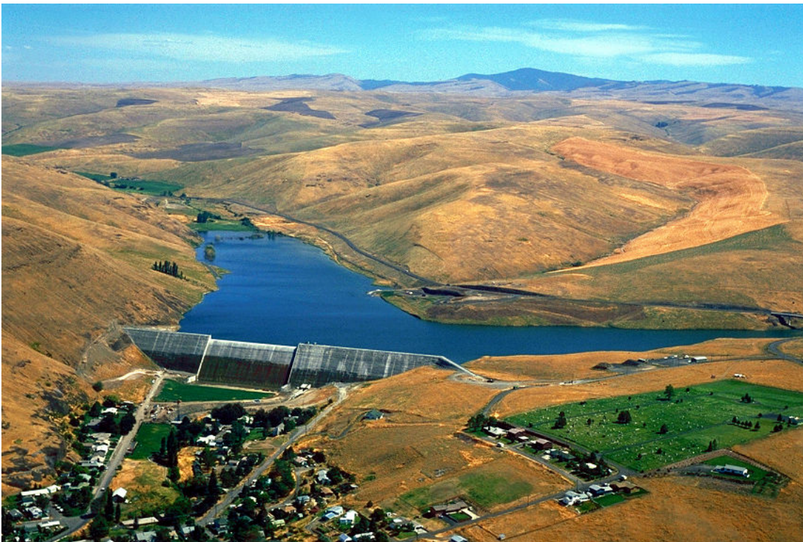
Figure 1–8: The Willow Creek Dam, just outside of Heppner, Oregon. (Source: U.S. Army Corps of Engineers/Creative Commons (Public Domain)/ https://commons.wikimedia.org/wiki/File:USACE_Willow_Creek_Dam_Oregon.jpg )
