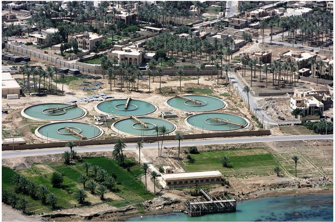
Figure 1-14: A water treatment facility in Ramadi, Iraq. (Source: Jeremy M. Giacomino, United States Marine Corps/Creative Commons (Public Domain)/ https://commons.wikimedia.org/wiki/File:Water_treatment_plant_in_Ramadi.jpg )
