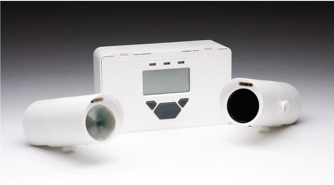
Figure 6-3: The transmitter (left), receiver (right), and control box (middle) of an end-to-end beam detector. (Source: Fire Fighting Enterprises (Depwaldrontoo)/Creative Commons (CC BY 3.0)/ https://commons.wikimedia.org/wiki/File:Optical_beam_smoke_detector.jpg )
