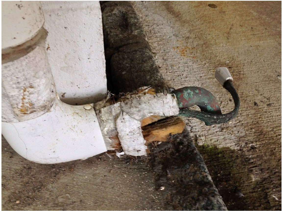
Figure 4-12: A self-regulating heat tracing wire is run alongside a copper pipe to provide freeze protection. (Source: z22/Creative Commons (CC BY-SA 3.0)/ https://commons.wikimedia.org/wiki/File:Self-regulating_heat_tracing_tape.jpg )
