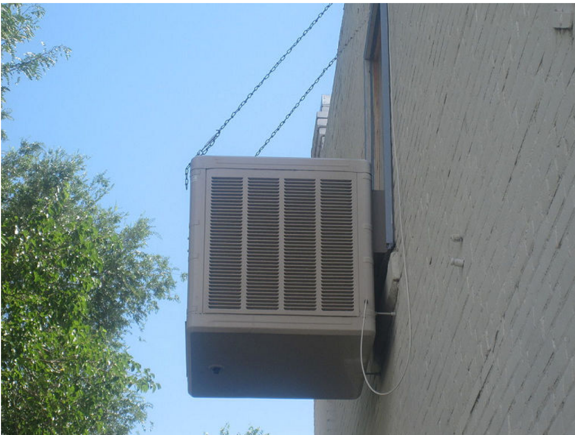
Figure 4-14: An evaporative cooler hangs off the side of the building in Colorado, where drier conditions allow it to be used as a source of cool air. (Source: Billy Hathorn/Creative Commons (CC BY-SA 3.0)/ https://commons.wikimedia.org/wiki/File:Evaporative_cooler,_CO,_IMG_5681.JPG )
