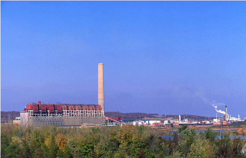
Figure 1-10: The Johnsonville Fossil Plant near Waverly, Tennessee produces enough electricity through coal combustion to supply 800,000 homes. (Source: Tennessee Valley Authority/Creative Commons (Public Domain/ https://commons.wikimedia.org/wiki/File:Johnsonville_fossil_plant.jpg ))
