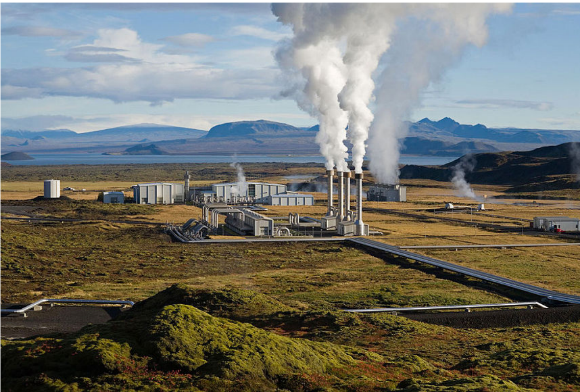
Figure 2–20: Steam rises from the stacks of a geothermal power plant in Iceland. (Source: Gretar Ivarsson/Creative Commons (Public Domain)/ https://commons.wikimedia.org/wiki/File:NesjavellirPowerPlant_edit2.jpg )
