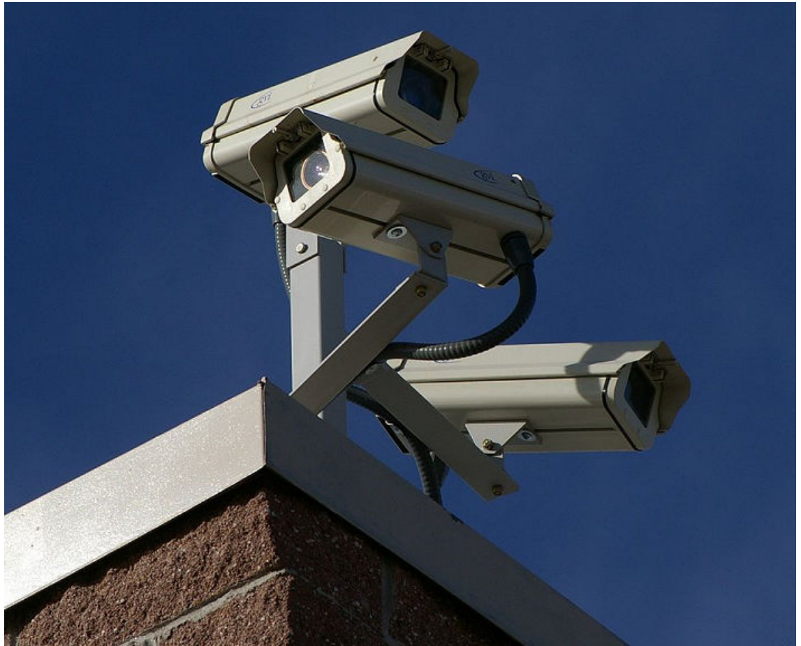
Figure 8–8: Surveillance cameras monitor and record the actions happening outside of a facility. (Source: Hustvedt/Creative Commons (CC BY-SA 3.0)/ https://commons.wikimedia.org/wiki/File:Three_Surveillance_cameras.jpg )
