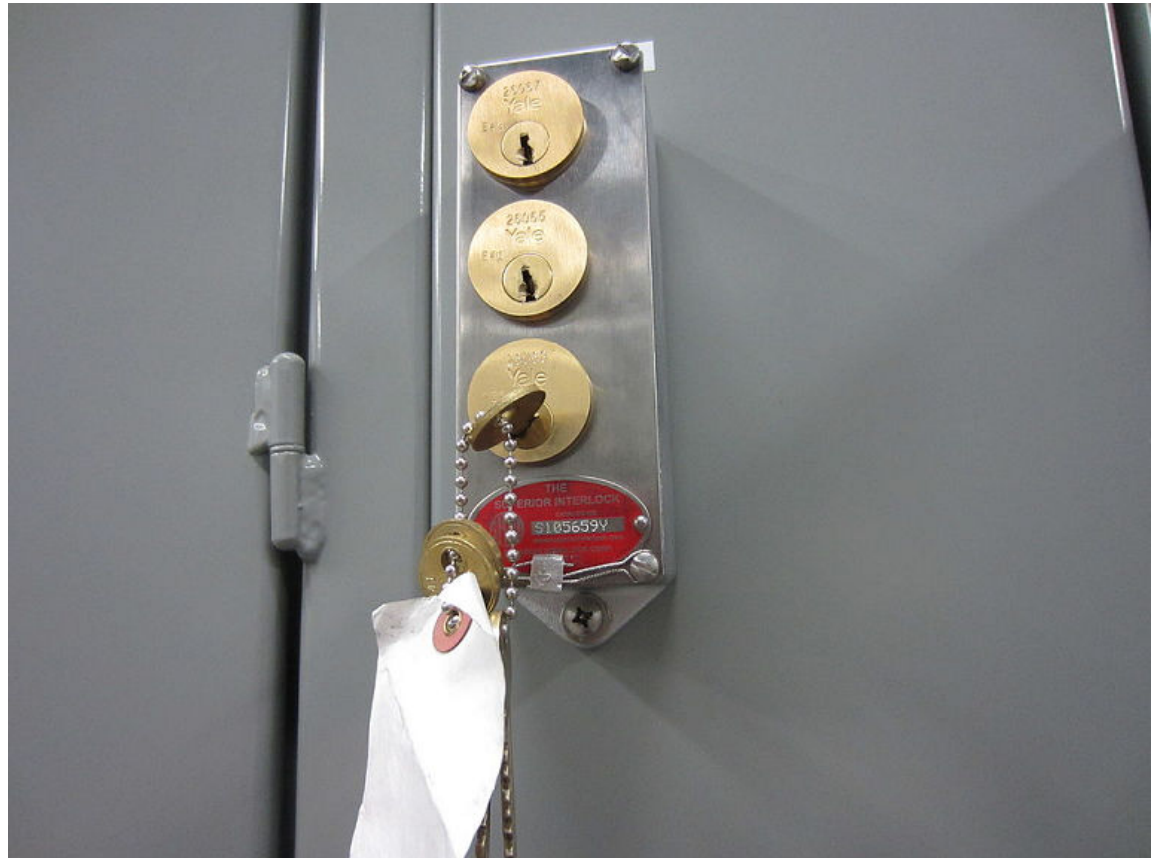
Figure 3–5: A Trapped Key Interlock. (Source: Wtshymanski/Creative Commons (CC BY-SA 4.0)/ https://commons.wikimedia.org/wiki/File:Trapped_key_interlock_transfer_block.JPG )
