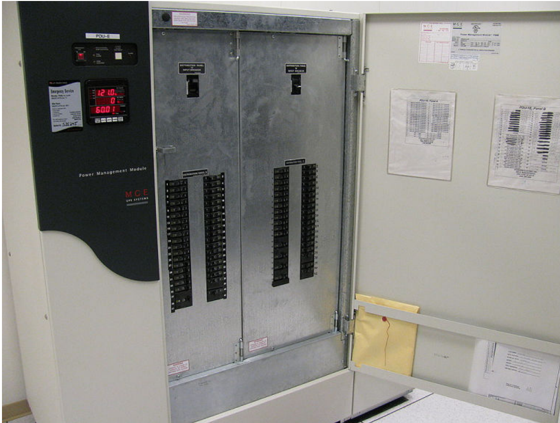
Figure 3–2: A cabinet PDU, shown with its door open, is designed to support a much larger-scale power distribution system. (Source: Robert.Harker/Creative Commons (CC BY-SA 3.0)/ https://commons.wikimedia.org/wiki/File:UPS_PDU_Open.jpg )
