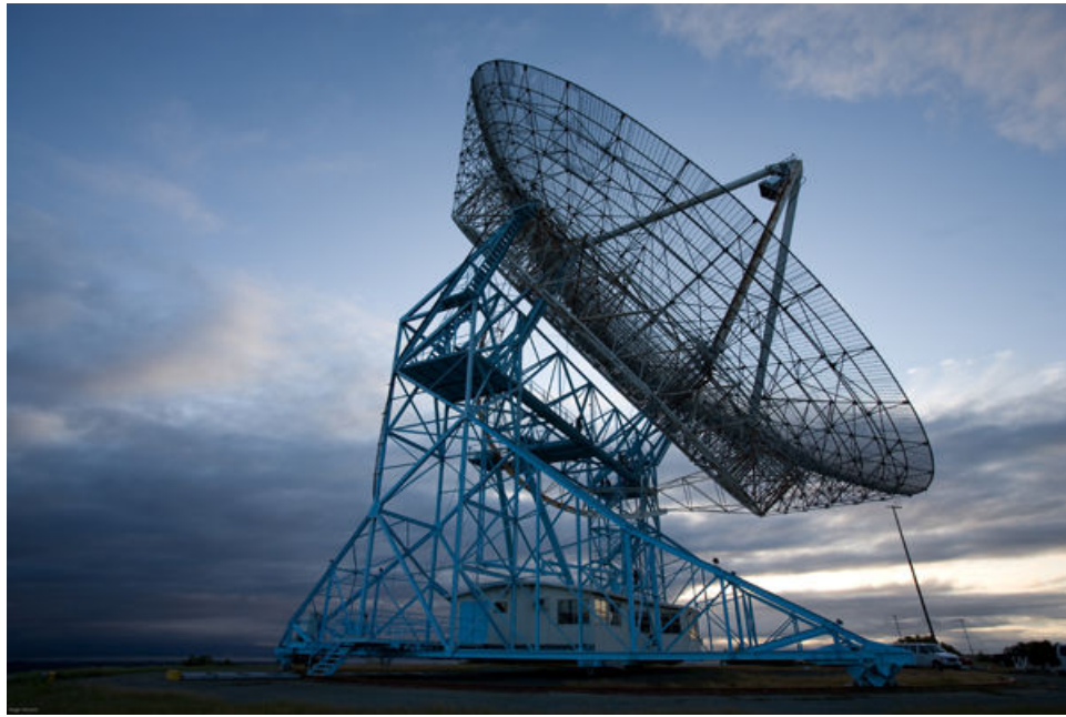
Figure 11–2: A radio communications antenna. (Source: SRI International/Creative Commons (CC BY-SA 3.0)/ https://commons.wikimedia.org/wiki/File:SRI_Dish_radio_antenna.jpg )
