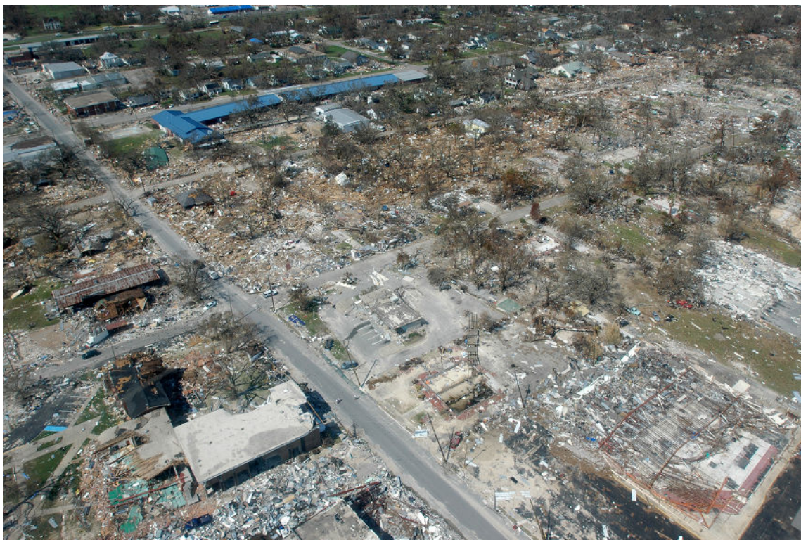
Figure 1-1: A hurricane—as evidenced by the damage seen here caused by Hurricane Katrina—can be a potential threat to MCO facilities. (Source: Federal Emergency Management Agency/Creative Commons (Public Domain)/ https://commons.wikimedia.org/wiki/File:Hurricane_katrina_damage_gulfport_mississippi.jpg )
