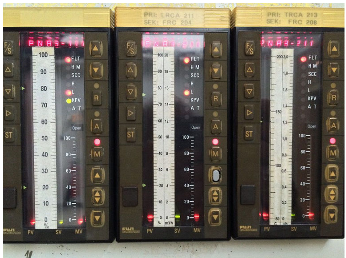
Figure 12–12: A Proportional–Integral–Derivative (PID) Controller can be used to determine the difference between a process variable and a desired set point, in order to adjust it appropriately. (Source: Bitjungle/Creative Commons (CC BY-SA 4.0)/ https://commons.wikimedia.org/wiki/File:Industrial_PID_controllers_-_front_display.jpg )
