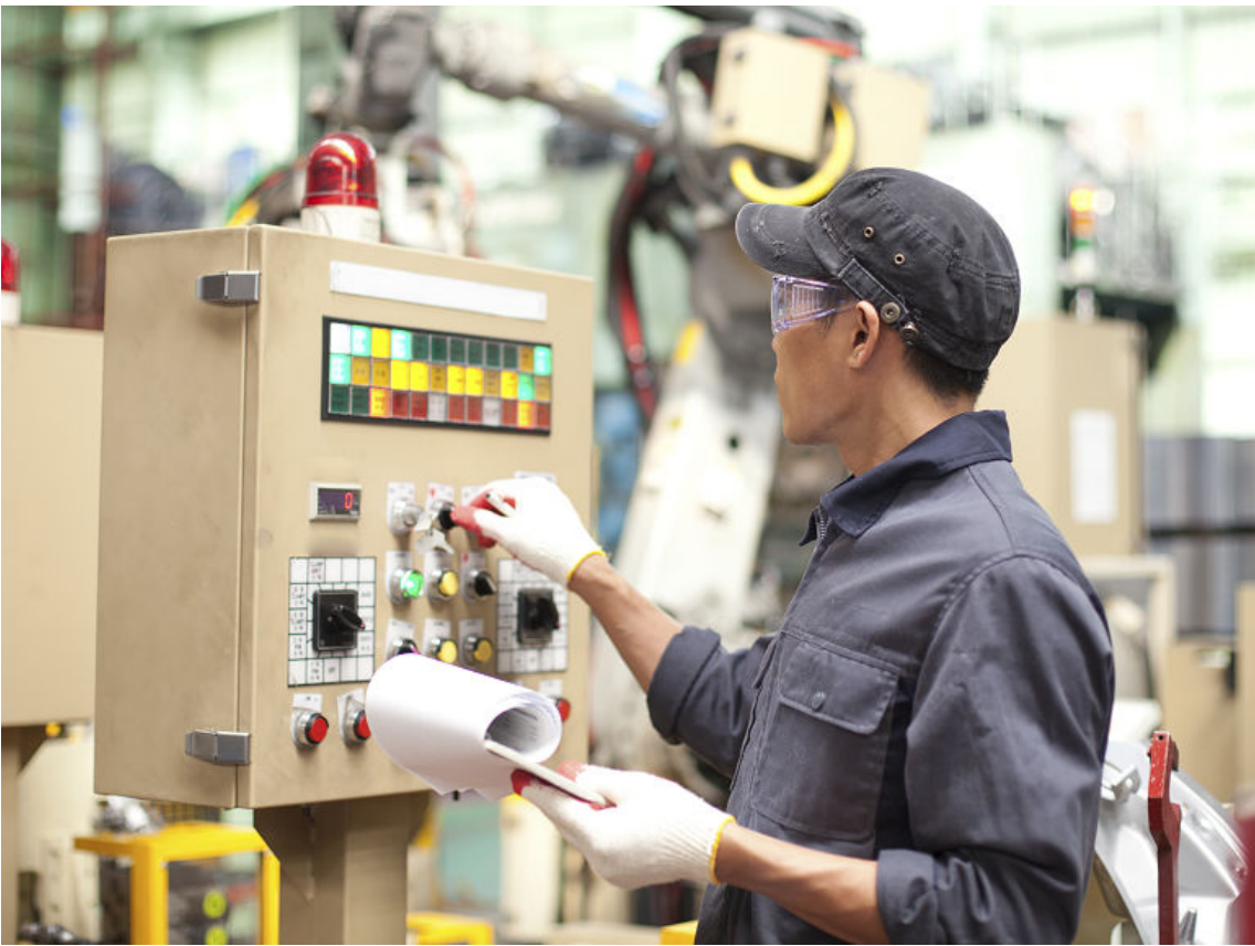
Figure 13-6: An engineer prepares to shut off power to energized equipment in order to perform necessary change-related work. (Source: ndoeljindoel/iStock/Thinkstock)
