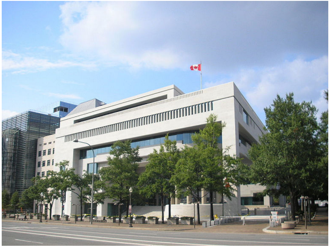
Figure 8–5: Large concrete planters act as a vehicle barrier to passing traffic in front of the Canadian Embassy in Washington, D.C. (Source: Gryffindor/Creative Commons (Public Domain)/ https://commons.wikimedia.org/wiki/File:Canadian_Embassy_DC_2007_002.jpg )
