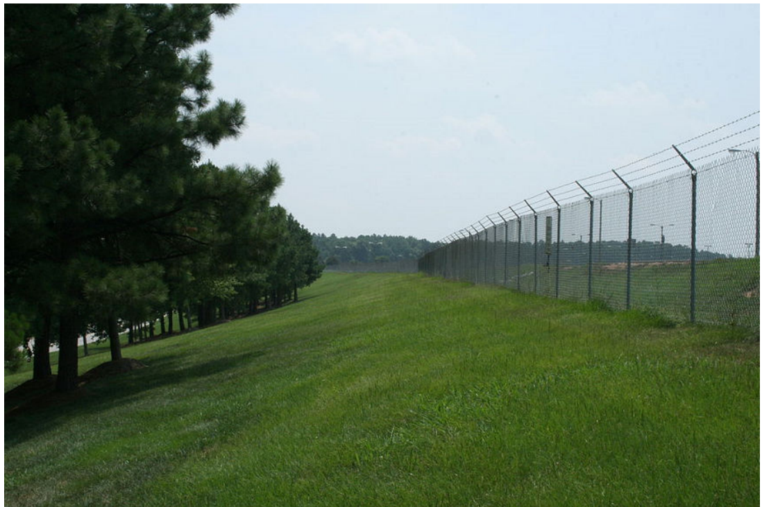
Figure 8–2: Fencing with the addition of barbed wire deters entry on to the property surrounding Raleigh–Durham International Airport. (Source: Ildar Sagdejev/Creative Commons (CC BY 3.0)/ https://commons.wikimedia.org/wiki/File:2008-07-30_Fence_along_Commerce_Blvd_at_RDU.jpg )
