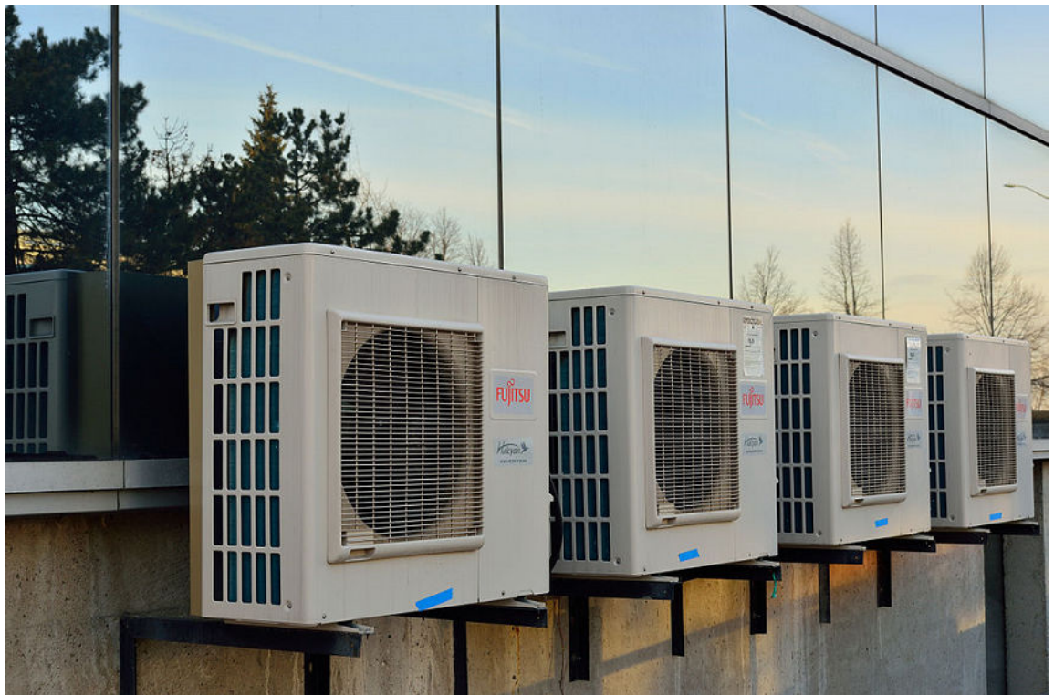
Figure 4-3: Air conditioning units provide cooling and humidity control for an office building. (Source: Raysonho/Creative Commons (Public Domain)/ https://commons.wikimedia.org/wiki/File:ACFujitsu.jpg )
