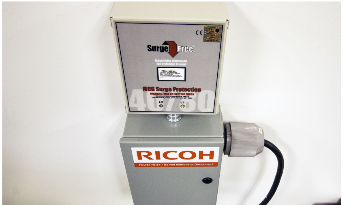
Figure 3–12: A TVSS surge protector in a printing and distribution space. (Source: Logical Operations for NCMCO)
