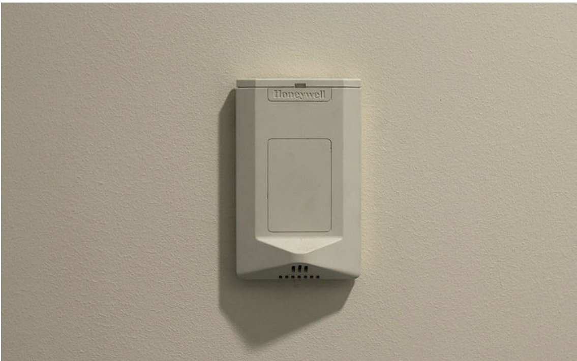
Figure 4–4: An electronic hygrometer monitors the amount of humidity in the air for an occupied space. (Source: Guillaume Piolle/Creative Commons (CC BY 3.0)/ https://commons.wikimedia.org/wiki/File:Honeywell_device.jpg )
