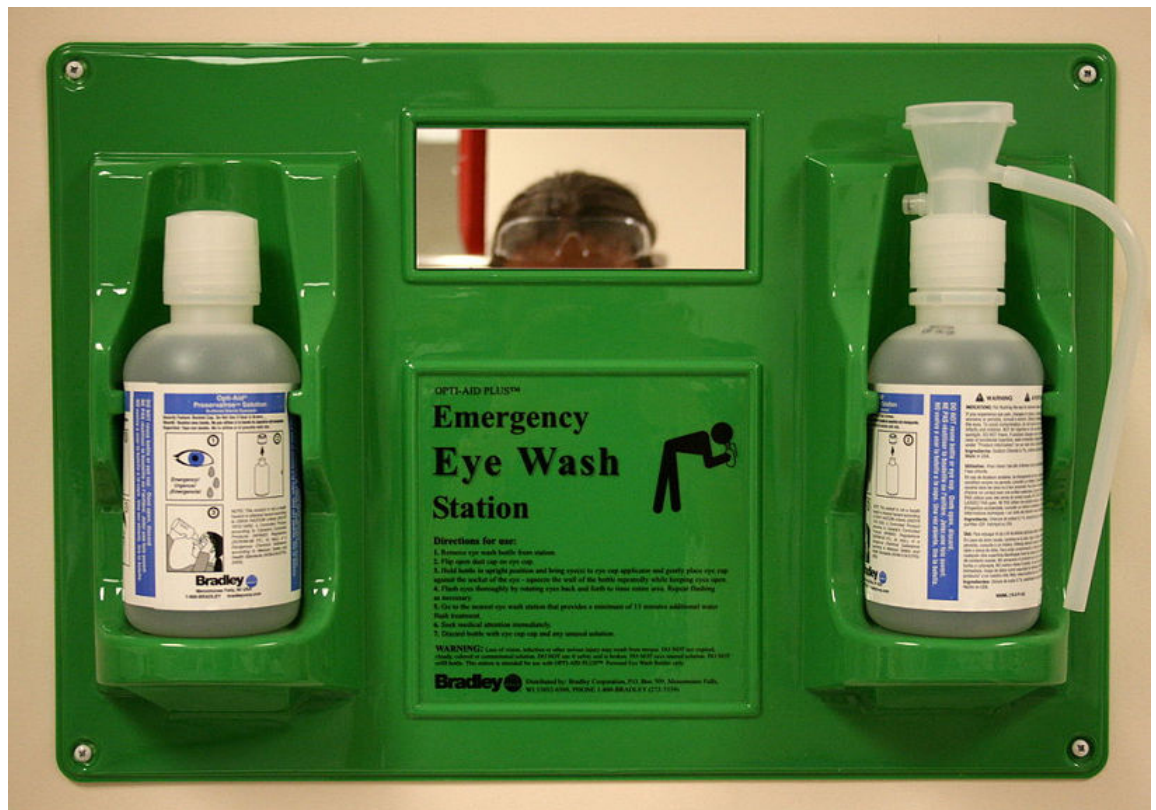
Figure 7-2: An eye washing station. (Source: Ildar Sagdejev/Creative Commons (CC BY-SA 3.0)/ https://commons.wikimedia.org/wiki/File:2008-07-02_Eye_wash_station.jpg )
