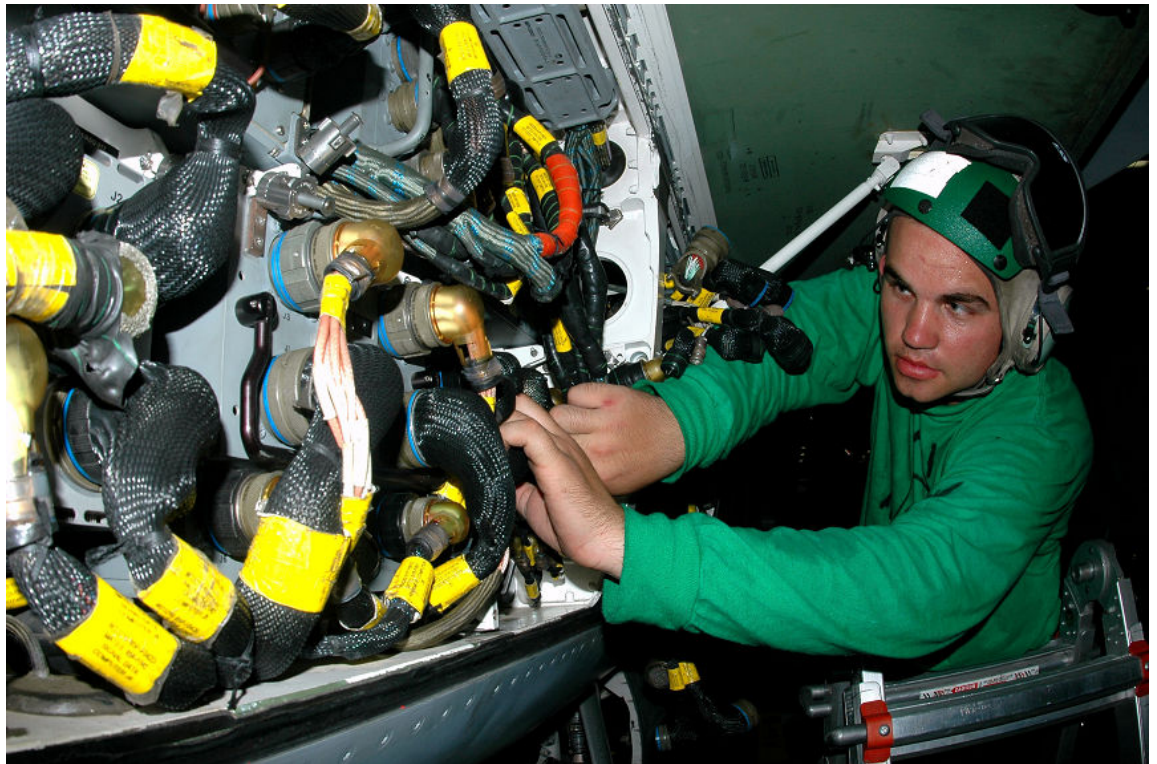
Figure 1–15: An Avionics Electronic Technician with the U.S. Navy installs a flight control computer in a fighter jet. (Source: United States Navy/Creative Commons (Public Domain)/ https://commons.wikimedia.org/wiki/File:US_Navy_070424-N-9760Z-020_Aviation_Electronics_Technician_3rd_Class_Patrick_Beckwith,_assigned_to_the_Top_hatters_of_Strike_Fighter_Squadron_(VFA)_14,_works_on_installing_a_flight_control_computer_in_a_F-A-18E_Super_Hornet.jpg )
