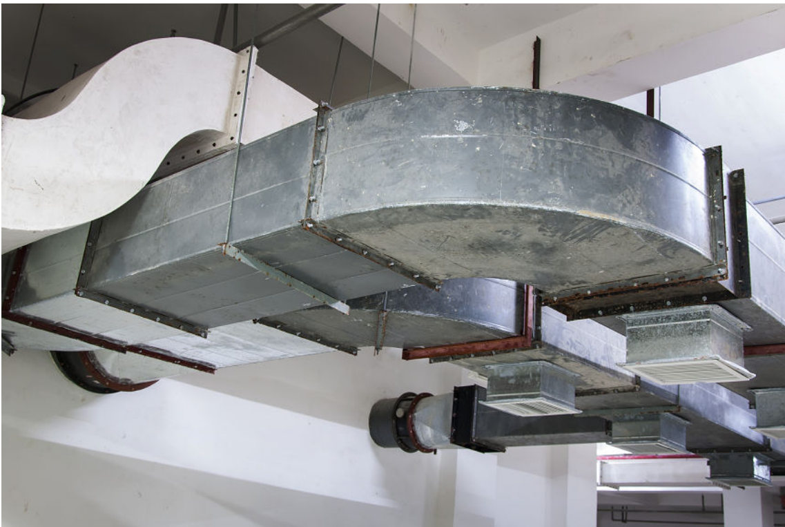
Figure 4-17: Ductwork transports conditioned air within a facility. (Source: Jeff_Hu/iStock/Thinkstock)
