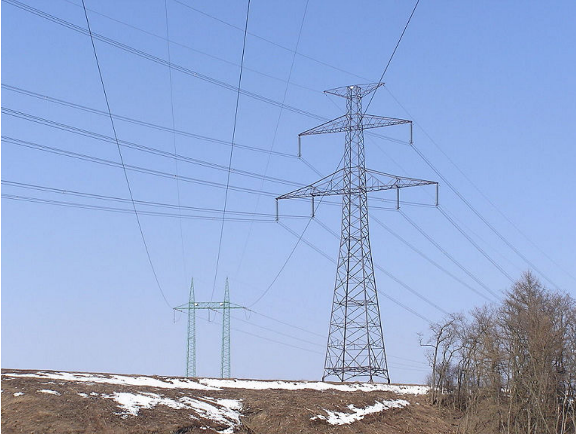
Figure 2-1: Power lines provide the type of electricity we are most familiar with: the kind that provides power to our homes and businesses. (Source: Jan Dudik/Creative Commons (Public Domain)/ https://commons.wikimedia.org/wiki/File:Lec06m76.JPG )
