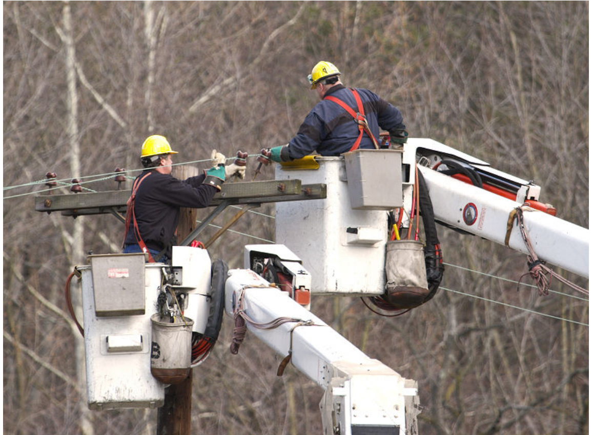
Figure 13–7: Two linemen follow the double custody switching protocol while performing maintenance on a power line. (Source: rpernell/iStock/Thinkstock)
