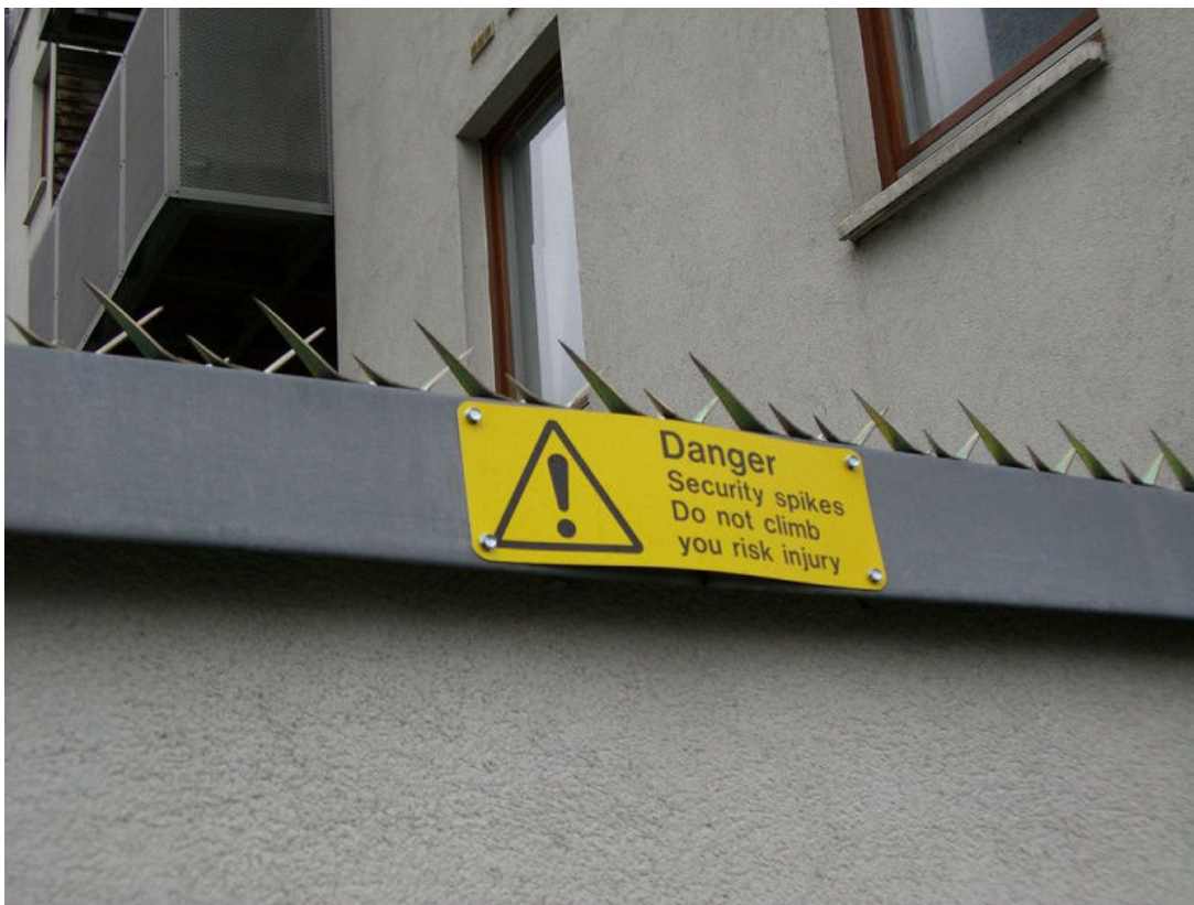
Figure 8-1: Both the sign and the spikes on this barrier wall indicate that unauthorized persons should not attempt to enter the secured space. (Source: Edward/Creative Commons (Public Domain)/ https://commons.wikimedia.org/wiki/File:Security_spikes_1.jpg )
