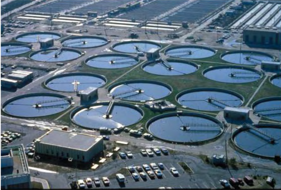
Figure 25.1 Sewage Treatment Plant (credit: "eutrophication&hypoxia"/flickr.com)
